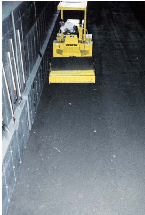
Figure 10. Compaction of subgrade soil.
