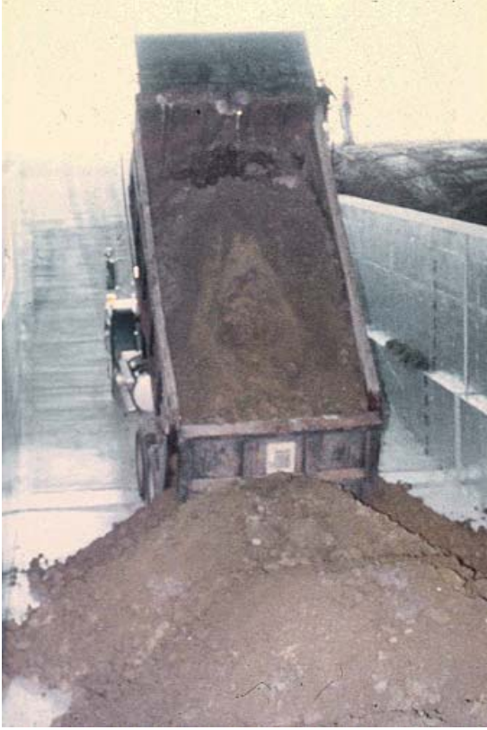
Figure 8. Placement of first lift in 701 test section.
