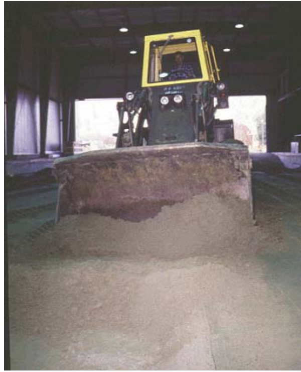
Figure 9. Grading of subgrade layer.
