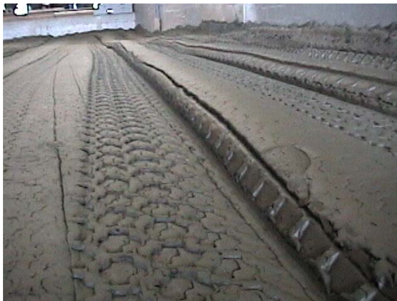
Figure 7b. Construction equipment tire marks on subgrade soil.
