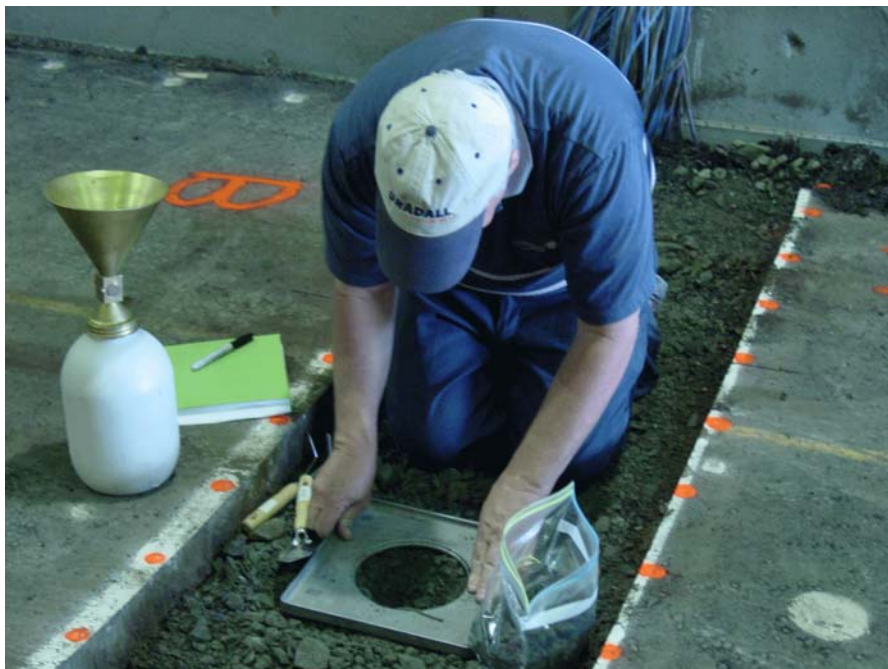
Figure 39a. Sand cone density measurements in the base course.
