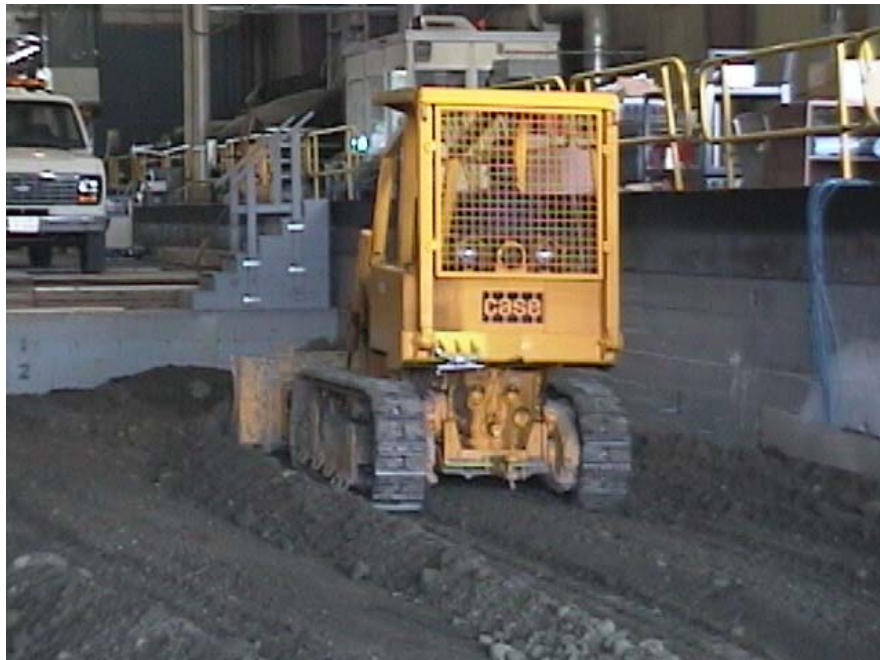
Figure 5. Bulldozer spreading and grading the subgrade soil.
