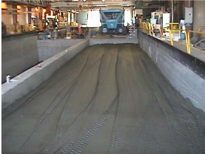
Figure 7a. Soft subgrade soil surface after rolling.
