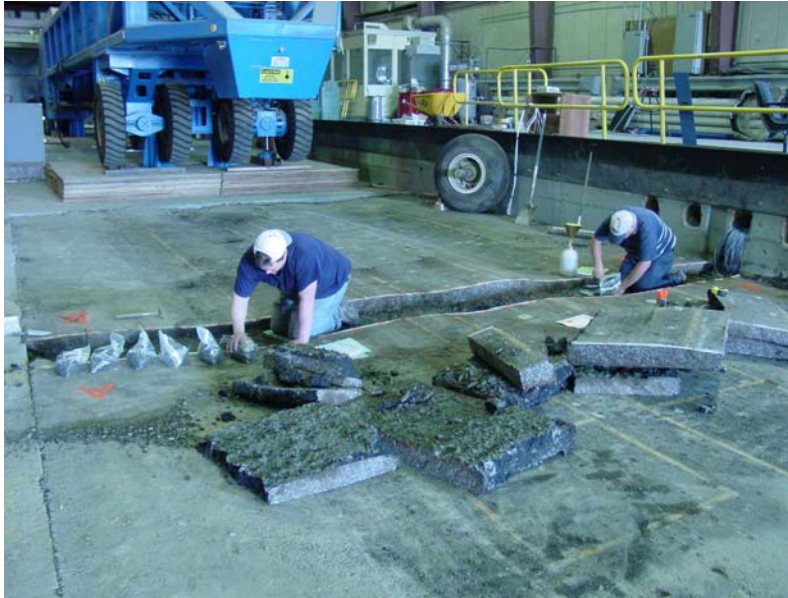
Figure 38. Forensic trenches across Test Windows 1, 2, and 3.
