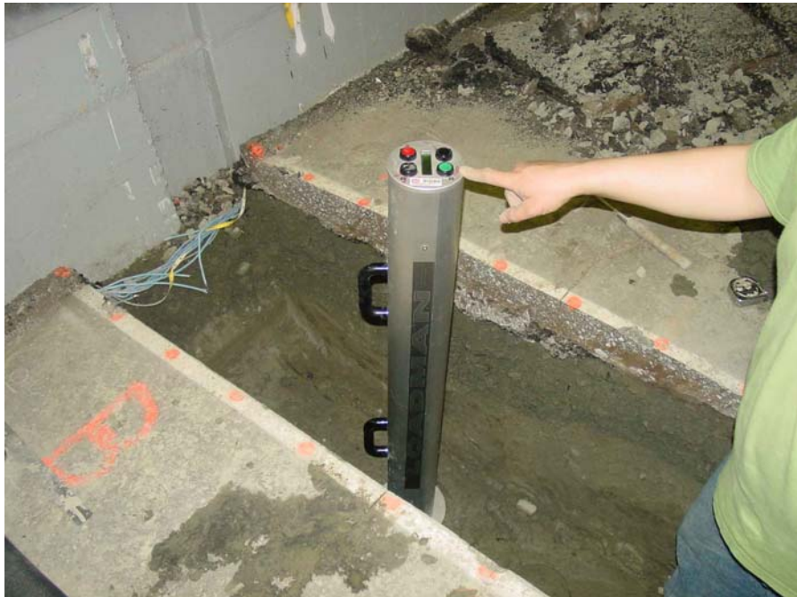
Figure 42a. Portable falling-weight deflectometer measurements in the trenches.
