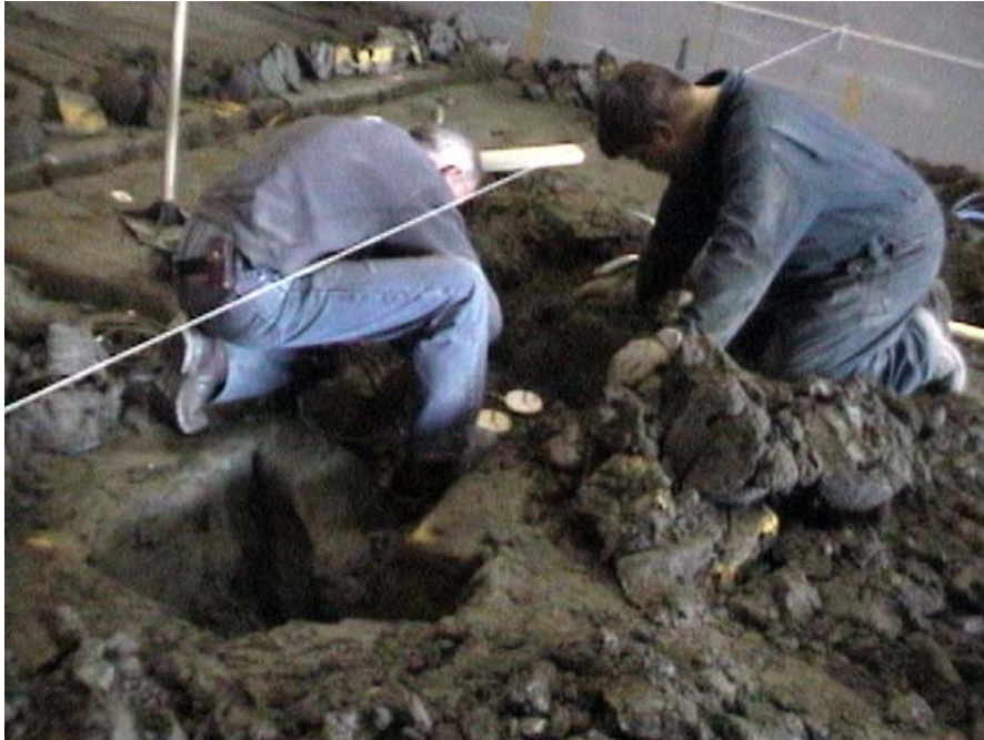
Figure 8. Installing sensors into the subgrade.
