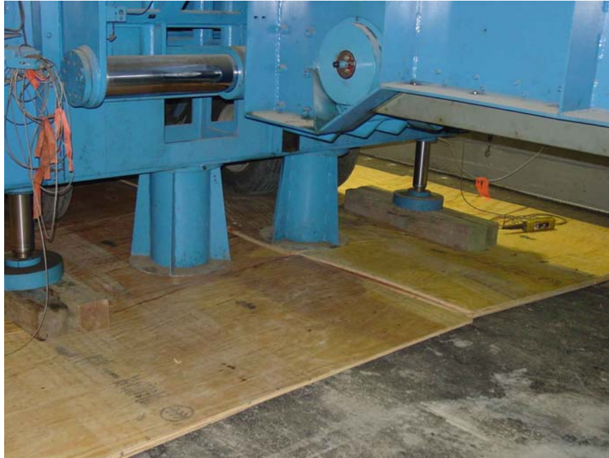
Figure 35. Pavement deformation at the HVS supports.
