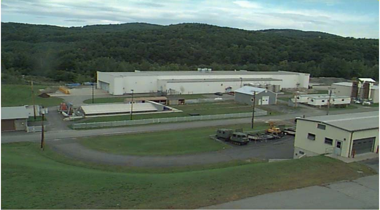
Figure A-1. Frost Effects Research Facility (FERF)
