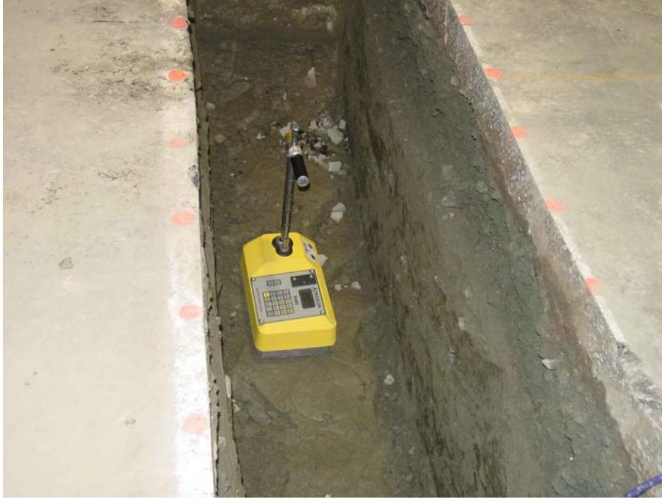
Figure 41a. Nuclear gauge density measurements in the trenches.
