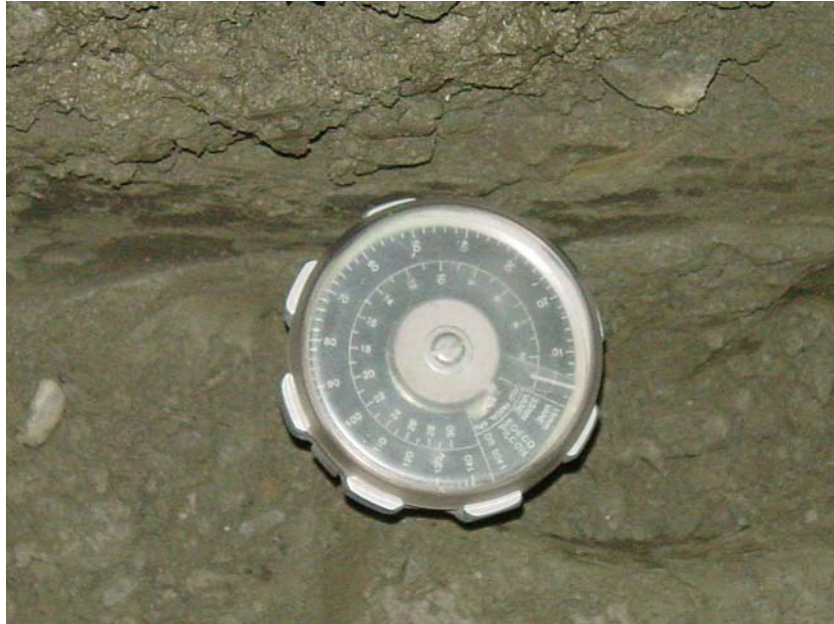
Figure 40a. Vane shear measurements in the subgrade at various depths.
