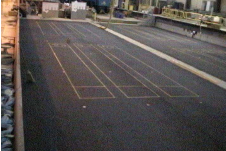
Figure 13. Constructed Test Section 706 with marked test windows.
