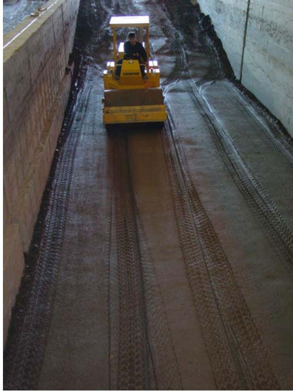
Figure 6. Roller compacting a subgrade A-6 soil layer at 22 percent gravimetric water content.
