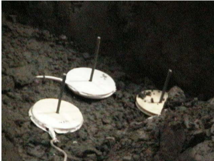
Figure 8. Emu coil sensors installed in the subgrade.
