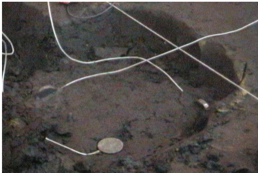
Figure 9. Dynatest® stress cells installed in the subgrade.
