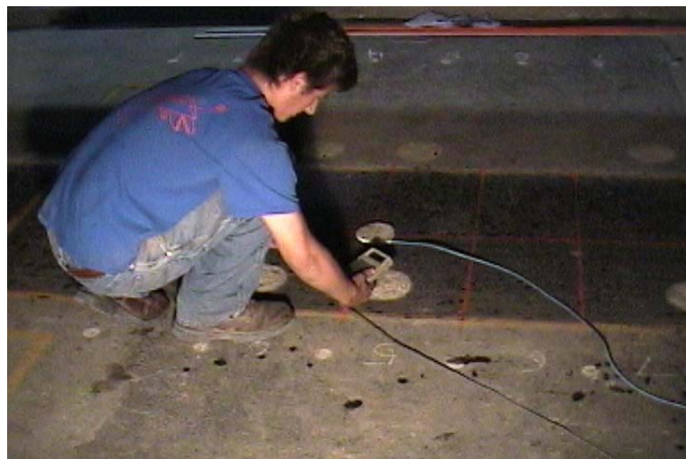
Figure 29. Measuring displacement between the AC surface and the top of the base course.
