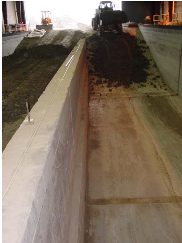
Figure 5. Empty test basin and start of subgrade building.
