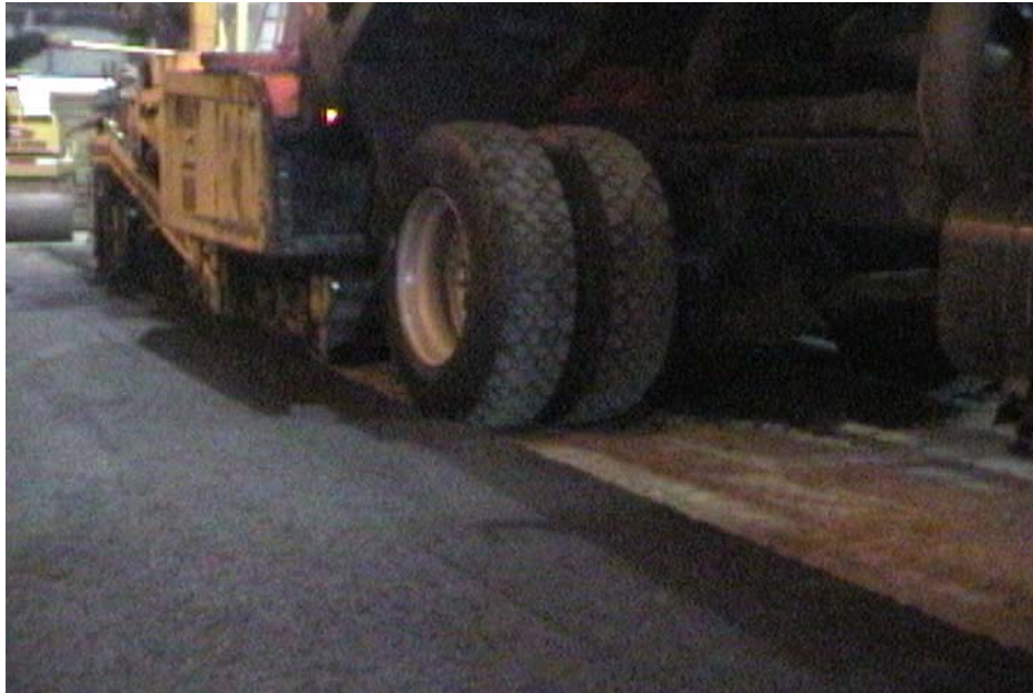
Figure 12. Paving of the test section.
