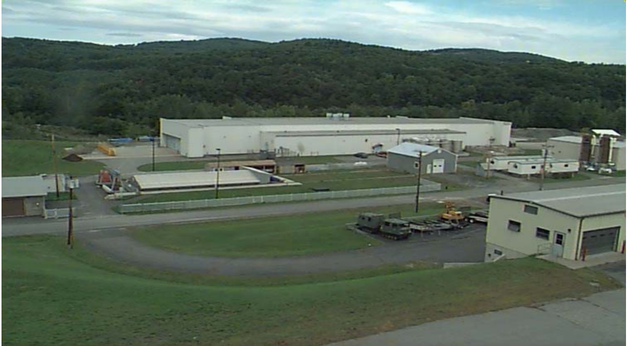
Figure A 1. Frost Effects Research Facility (FERF)
