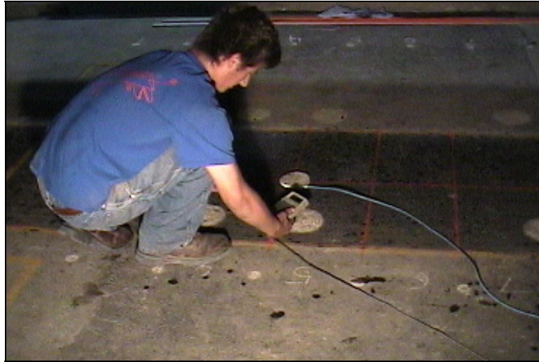
Figure 12. Measuring displacement between the AC surface and the top of the base course.
