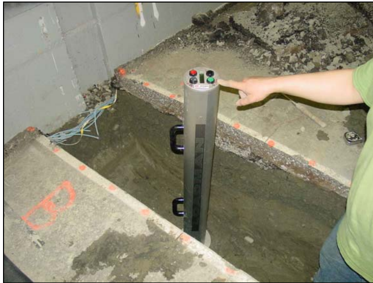
Figure 31. Portable falling-weight deflectometer measurements in the trenches.
