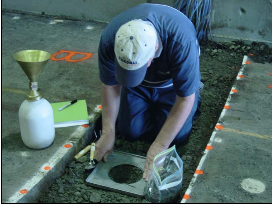
Figure 22. Sand cone density measurements in the base course.
