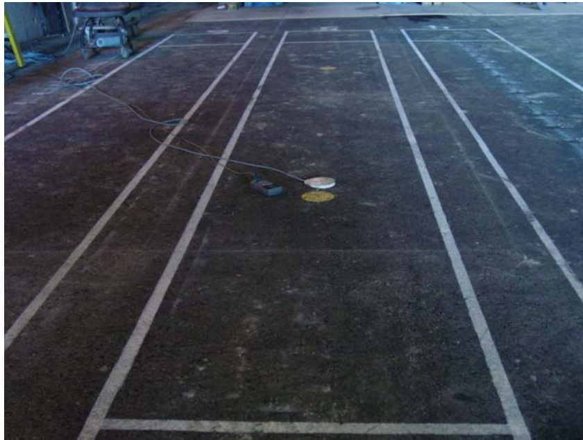
Figure 27. Test Window 711c5 before HVS traffic.
