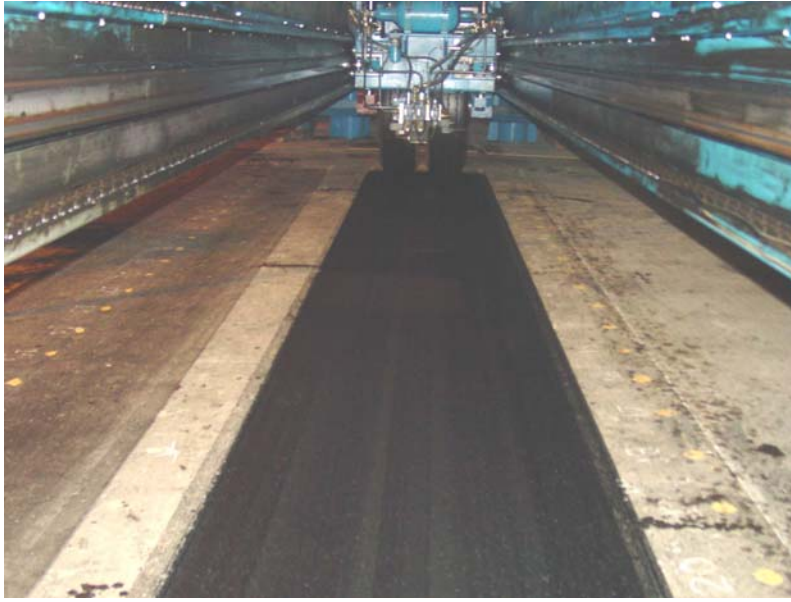
Figure 24. Test Window 711c2 at the end of HVS traffic.
