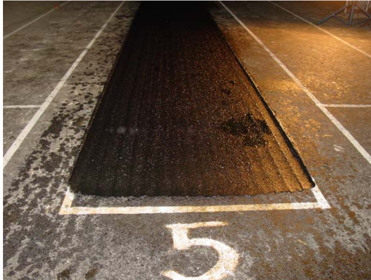
Figure 28. Test Window 711c5 at the end of HVS traffic.
