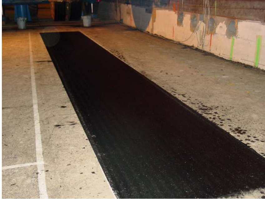
Figure 26. Test Window 711c3 at the end of HVS traffic.
