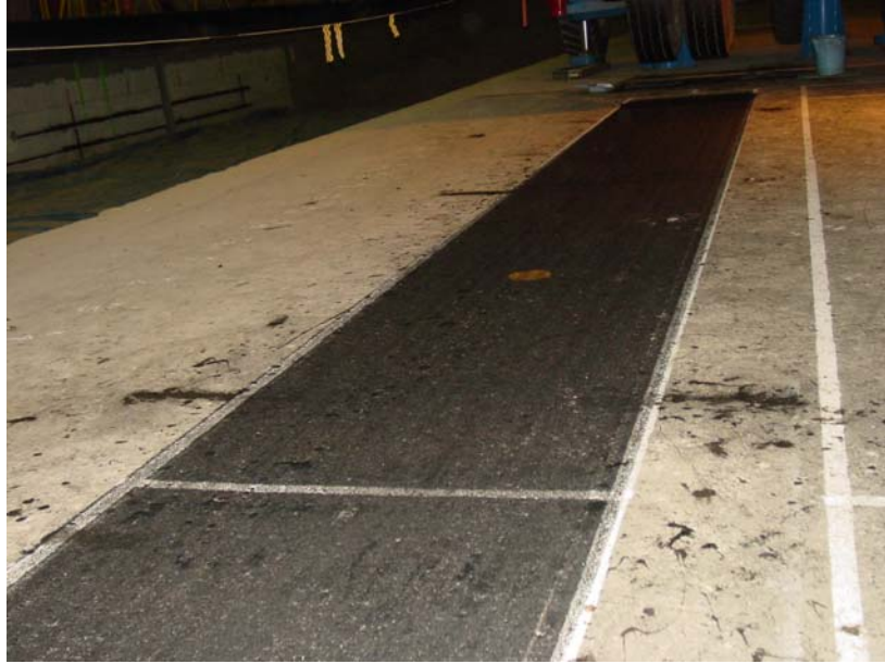
Figure 22. Test Window 711c1 at the end of HVS traffic.
