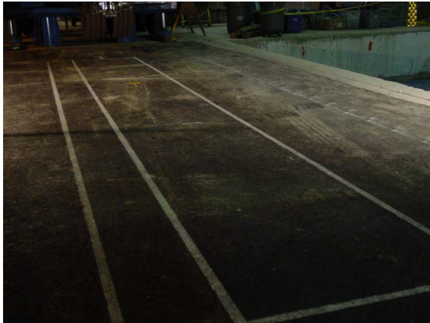
Figure 21. Test Window 711c1 before HVS traffic.
