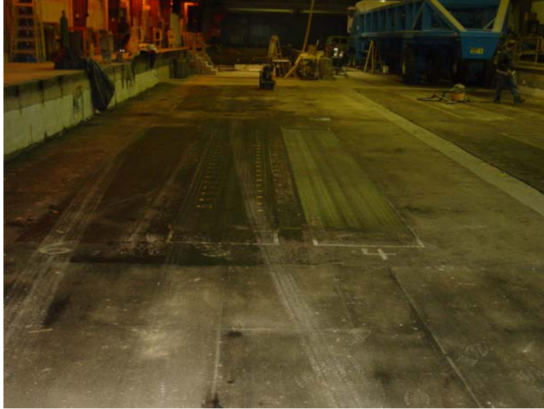
Figure 44. View of test section at the end of traffic tests.
