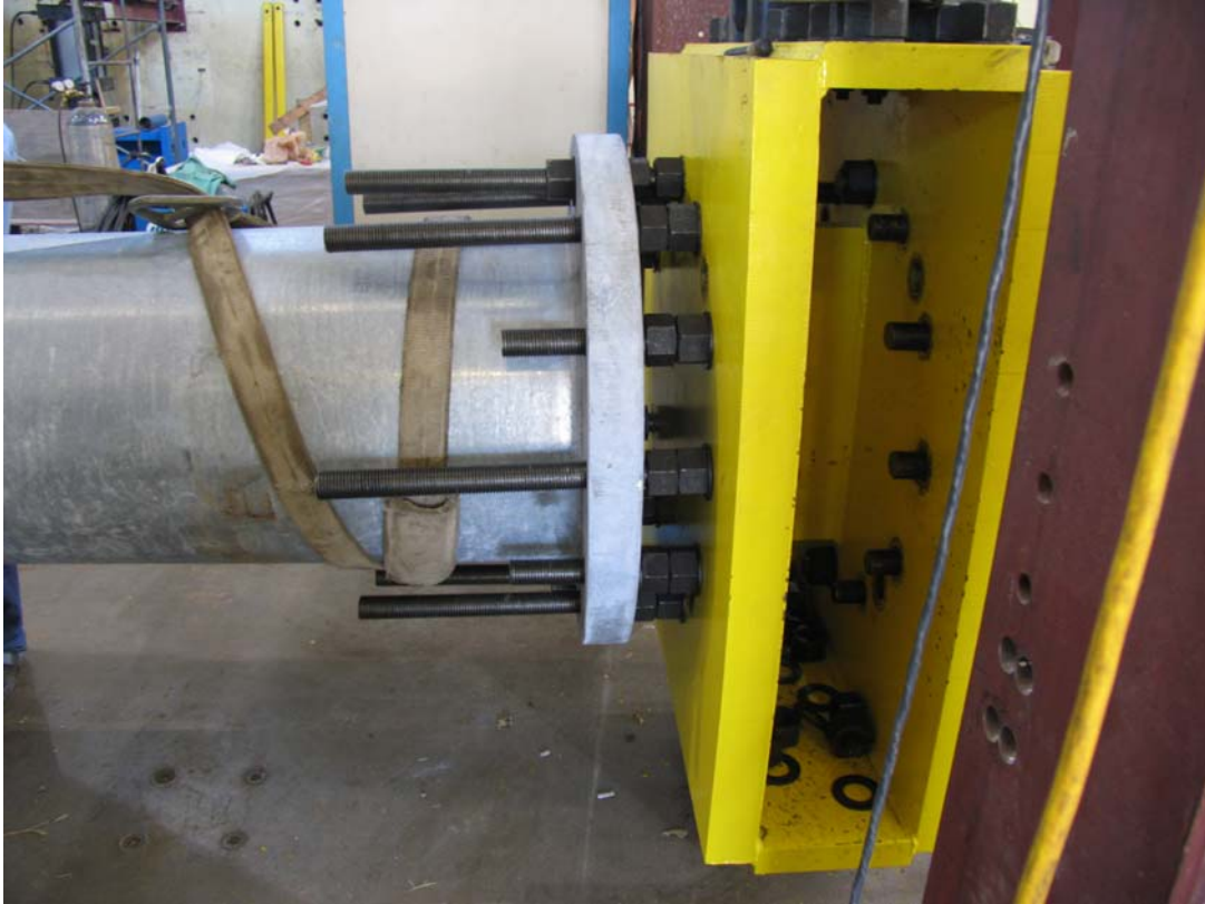
Figure 3: Leveling nuts used for base plate to loading box connection in large test setup
