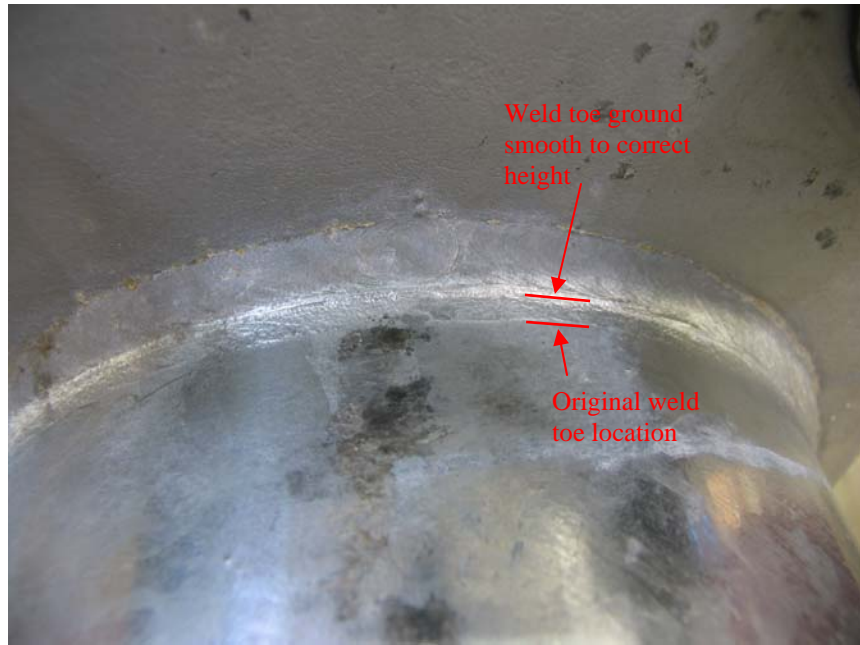
Figure 4: Grinding of the weld toe
