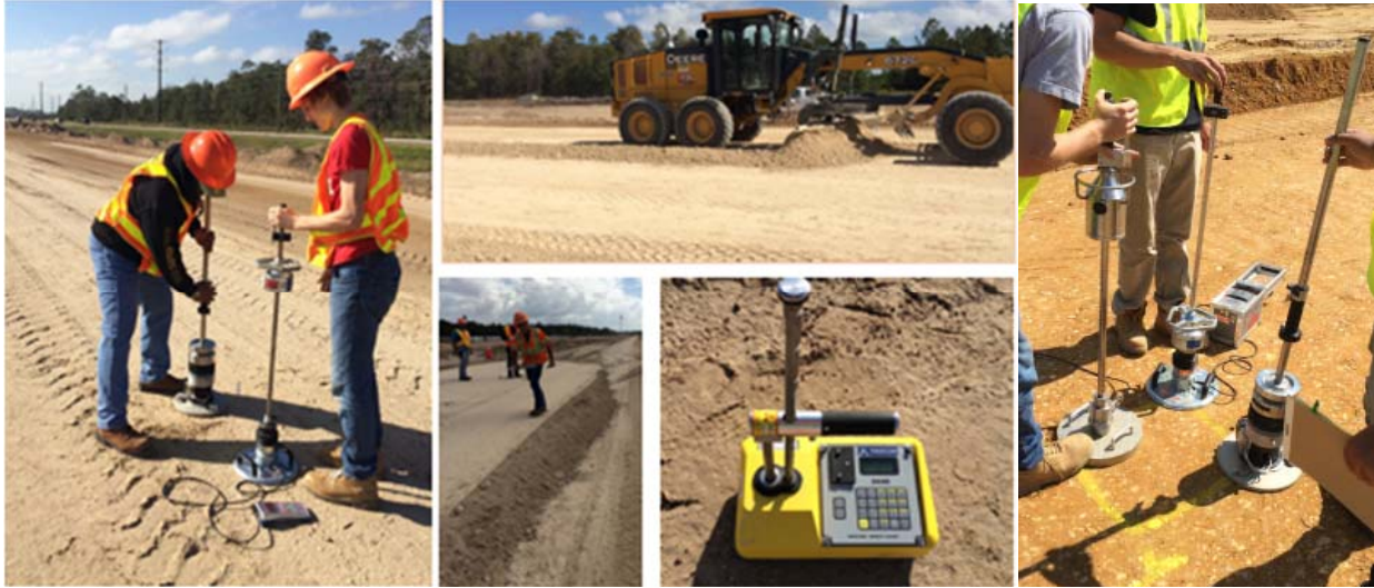
Figure 4-8. LWD and NDG testing on the subgrade and base after compaction
