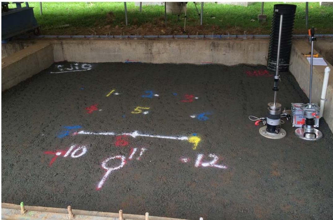
Figure 3-8. Test pit final compacted layer and LWD testing locations
