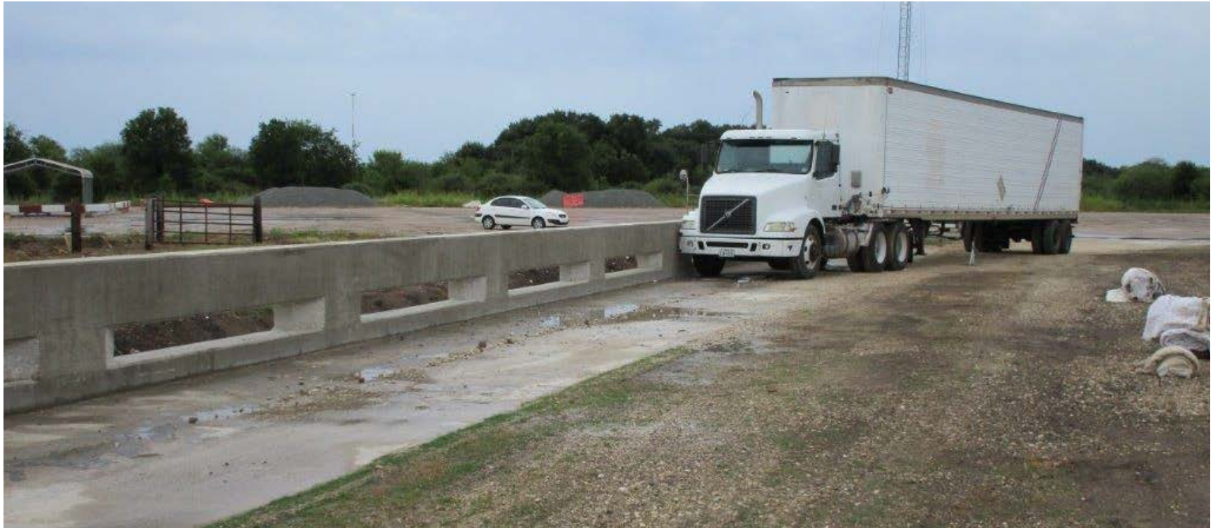
Figure 6. TTI TL-5 Open Concrete Bridge Rail System
