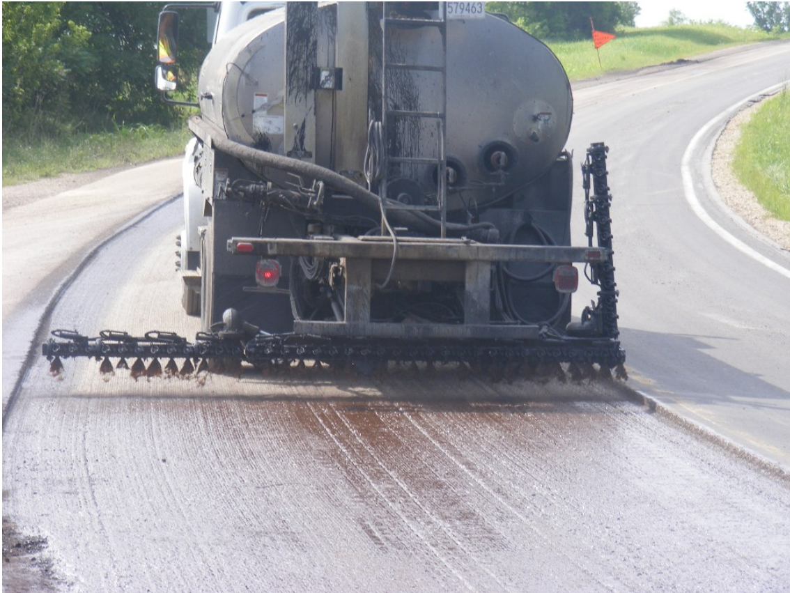
Figure 1.1: Tack Coat Application
