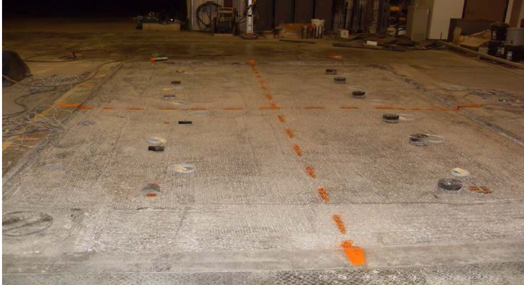
Figure 6.3: Installed Strain Gauges
