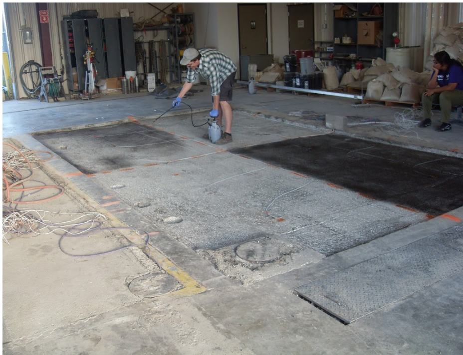
Figure 6.2: SS-1HP Tack Coat Application
