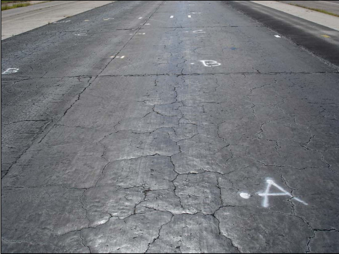
Figure 3. Skid Pad 2A.
