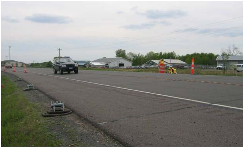
Figure 8.2 TIRTL Test Site
