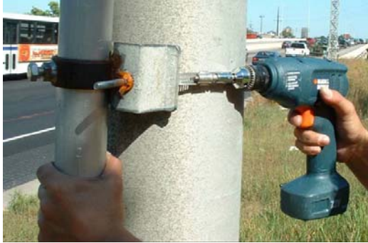
Figure 6.6 Round Light Pole Installation
