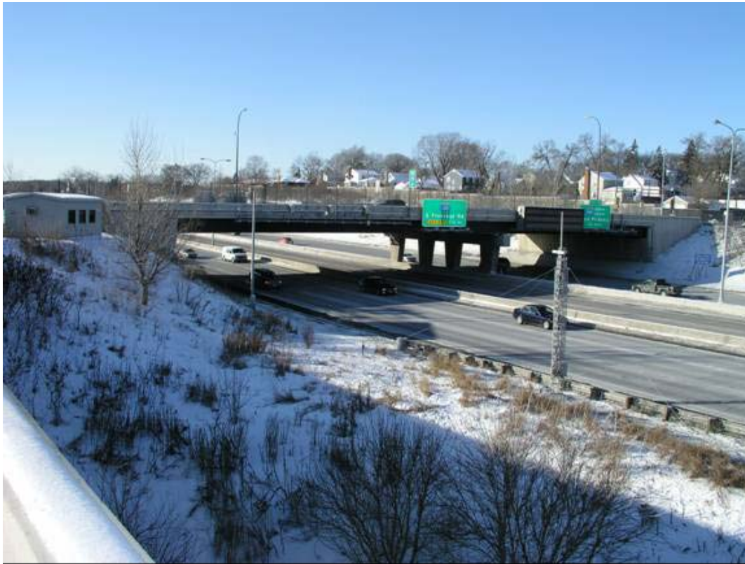
Figure 4.1: PNITDS Test Site
