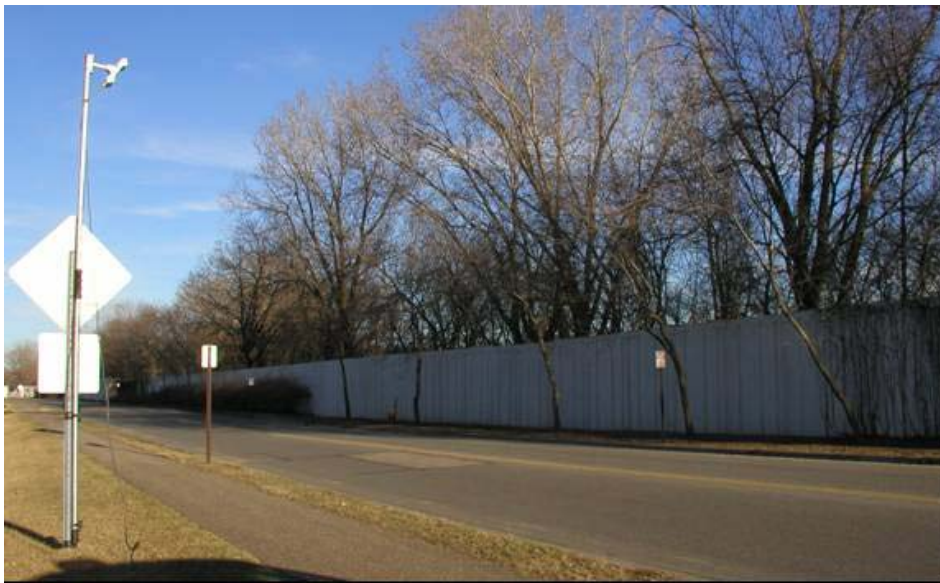
Figure 6.3 Test Site of a 2-lane Roadway with a Side Wall
