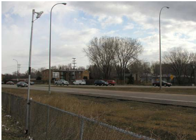
Figure 6.4 Test Site for Unparalleled Lanes at I-94 Exit Ramp
