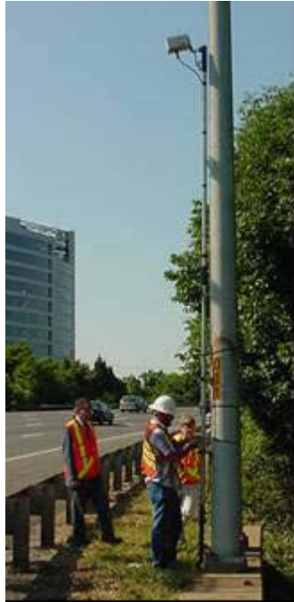
Figure 2.2: System Developed by Virginia DOT
