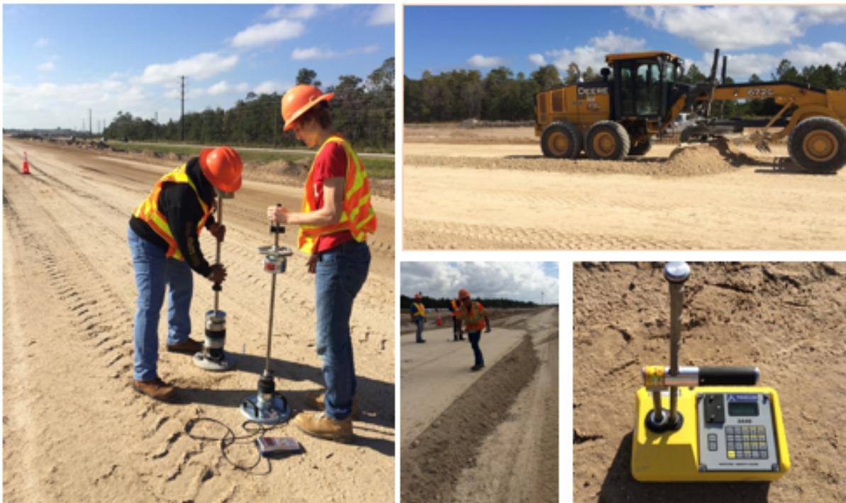
Figure 1- Jacksonville SR-23 project LWD and NDG testing on the subgrade and base after compaction
