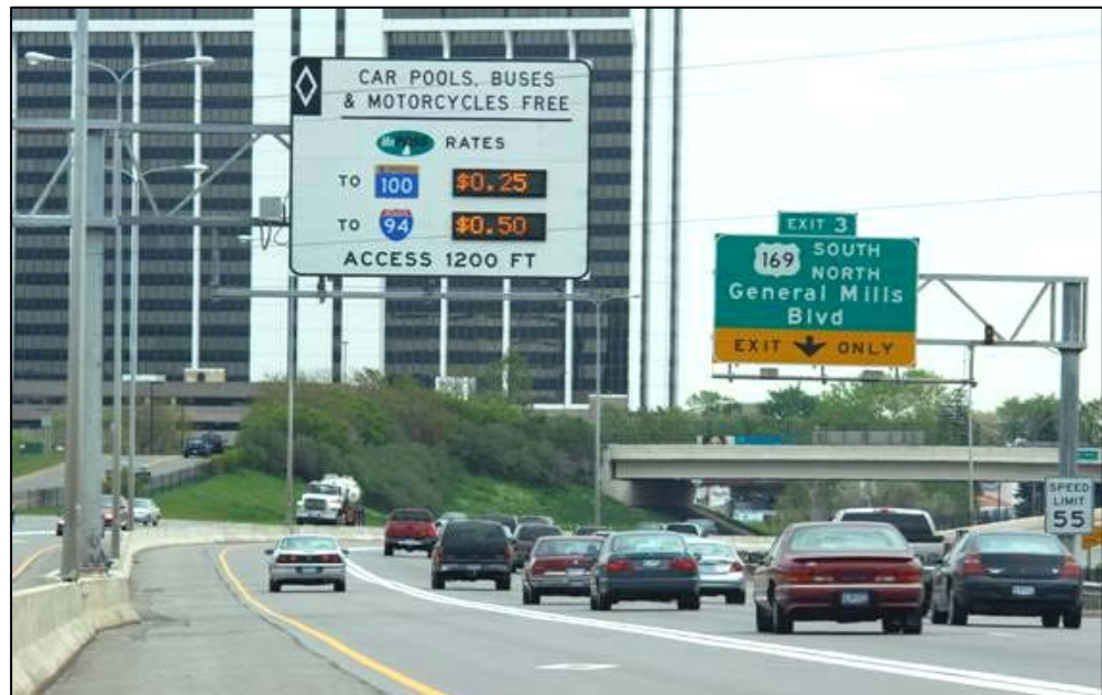
Figure 6-1. I-394 Express Lanes HOT Facility in Minneapolis.
