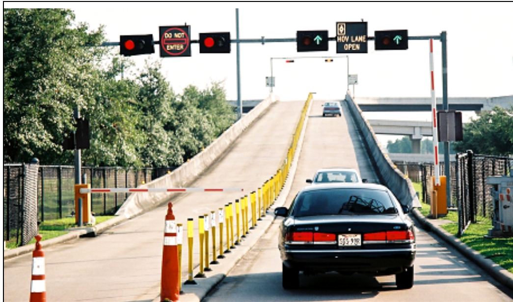
Figure 5-1. Operational Safety Treatments on Reversible HOV-Lane Park-and-Ride Ramp.
