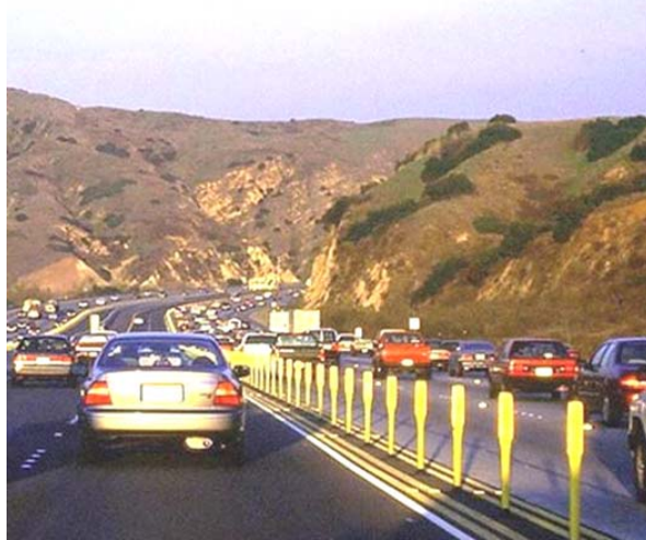
Figure 2-17. Flexible Tubular Markers Used to Reduce Buffer Violations
