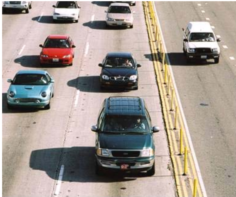
Figure 4-12. Flexible Tubular Markers Used to Reduce Buffer Violations.
