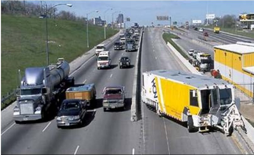
Figure 4-5. Transfer of Moveable Barrier for Contraflow Operations.
