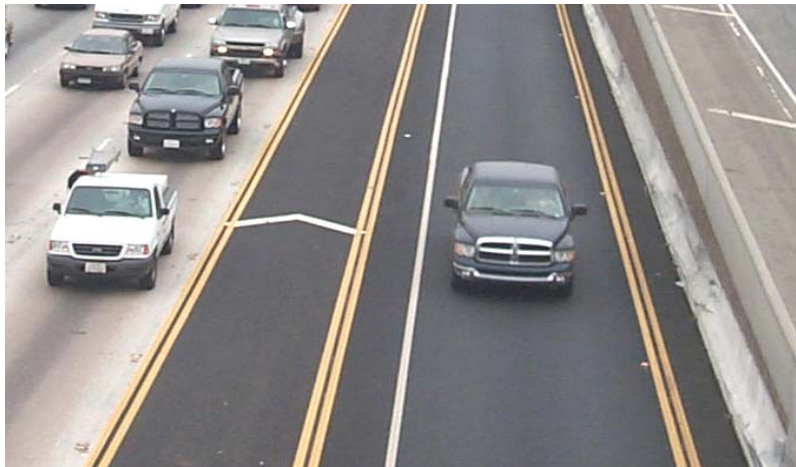
Figure 2-16. Concurrent Limited-Access HOV Lanes with Narrow (top), Medium (center), and Wide (bottom) Buffers
