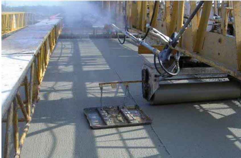
Figure 6.18 Fogging system mounted on the finishing bridge for LC-HPC 11
