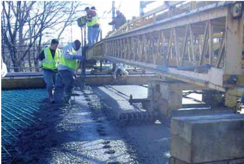
Figure 6.49 Inappropriate consolidation during construction of OP-p1
