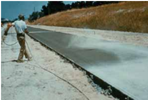
(c) Liquid membrane-forming compounds sprayed onto the surface are effective, economical moisture barriers for moist-curing concrete
