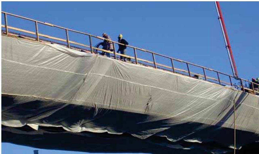
Figure 6.25 Deck and girders protection during curing in cold weather for LC-HPC 6
