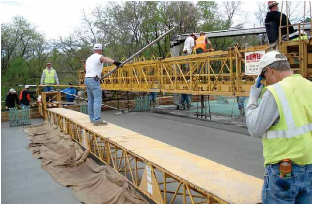
Figure 6.52 Burlap drag during construction of OP-p2
