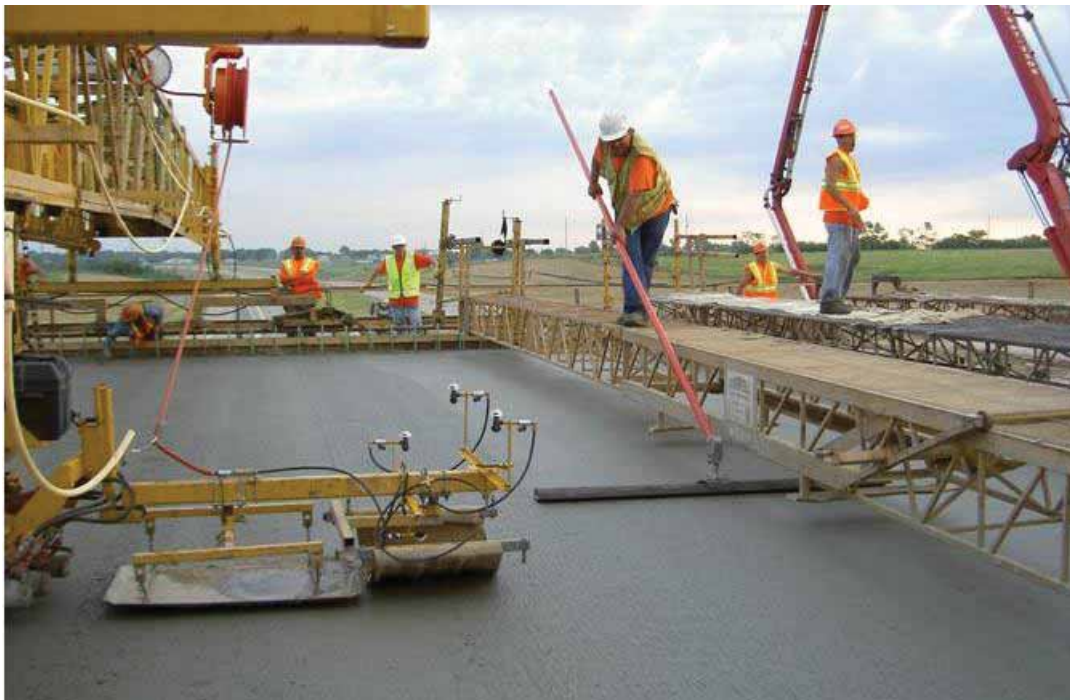
Figure 6.7 Finishing operation for LC-HPC 7
