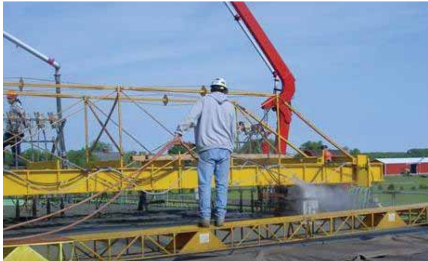
Figure 6.12 Hand-held fogging in LC-HPC 10
