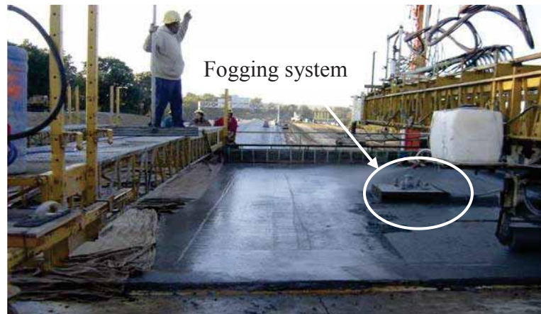
Figure 6.2 Fogging system mounted to the finishing bridge, followed by bullfloating operation
