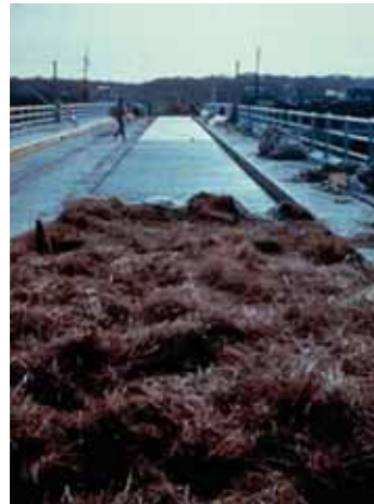
(d) Straw or hay is still used to insulate fresh concrete in freezing weather
