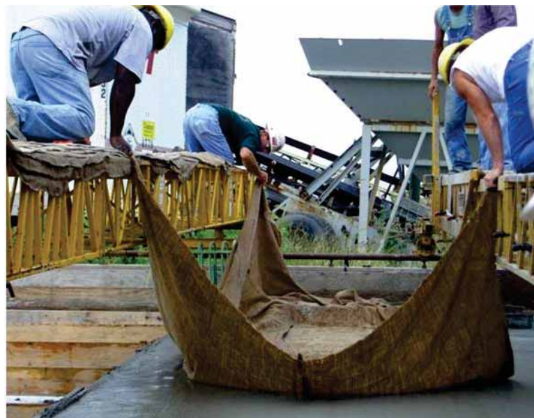
Figure 6.1 Burlap placement on the trial slab for LC-HPC 1
