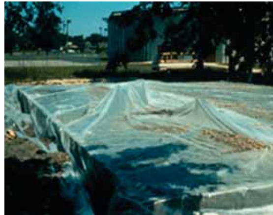
(b) Polyethylene sheets are effective, economical moisture barriers for moist-curing concrete
