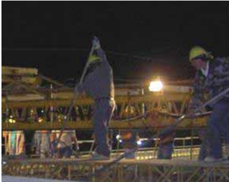
Figure 6.22 Bullfloating with two workers for LC-HPC 4-p1
