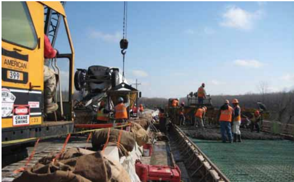
Figure 6.34 Placement with buckets for LC-HPC 12
