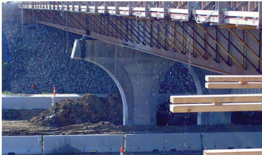
Figure 6.8 Water runoff the bridge when wetting the burlap on deck surface
