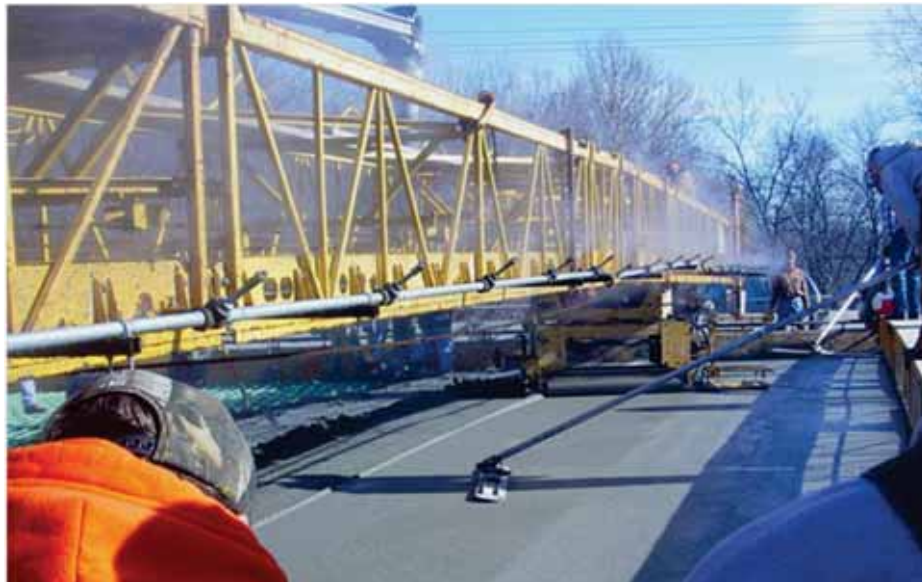
Figure 6.50 Bullfloating in longitudinal direction for OP-p1 (fogging was on)
