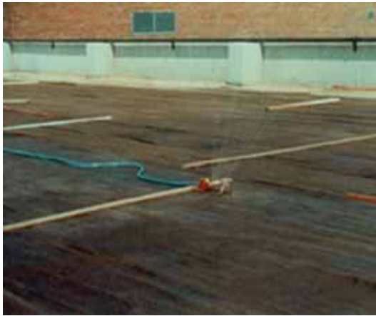
(a) Burlap kept saturated with water is an effective medium for moist-curing
