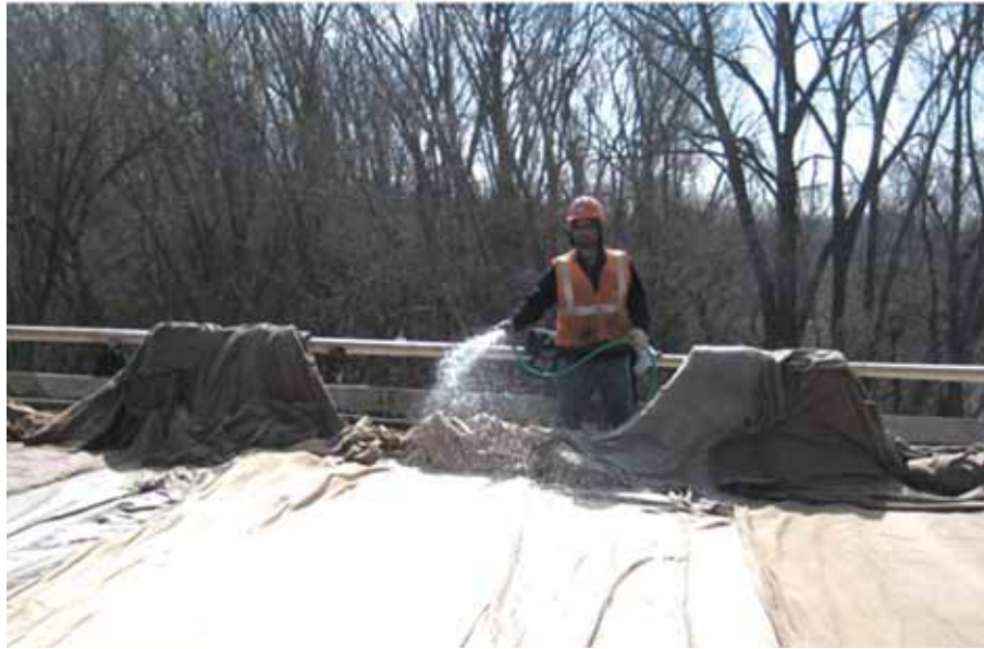
Figure 6.35 Burlap re-wetting for LC-HPC 12-p1
