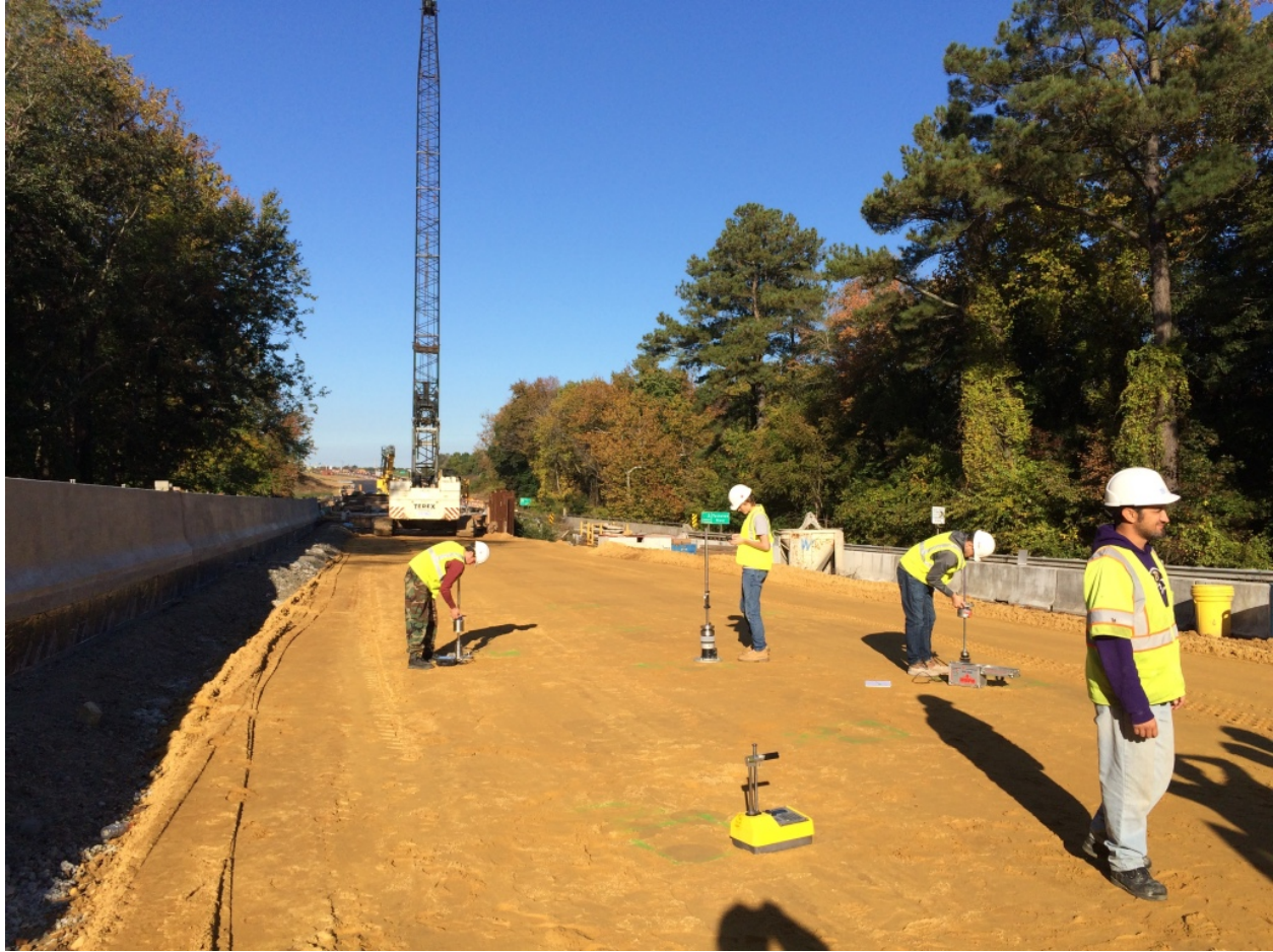
Figure 1- MD route 404 Subgrade LWD and NDG testing
