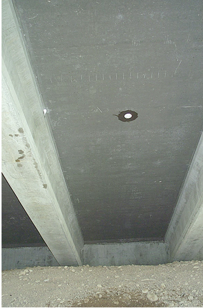
Figure 7: Beneath WB I-90 Slowway interchange after coring.
