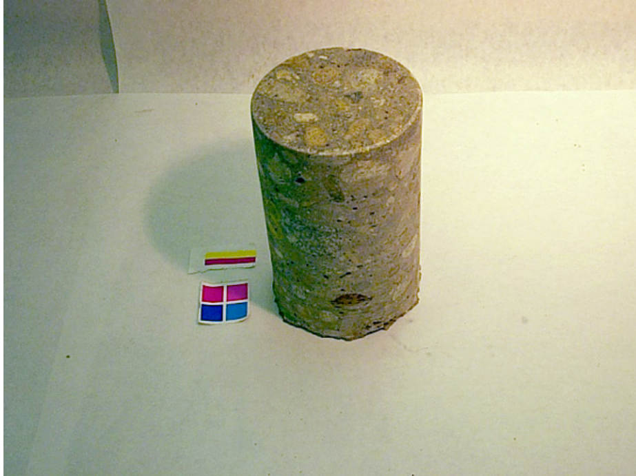
Figure 5: Core T-2, taken away from deteriorated area.
