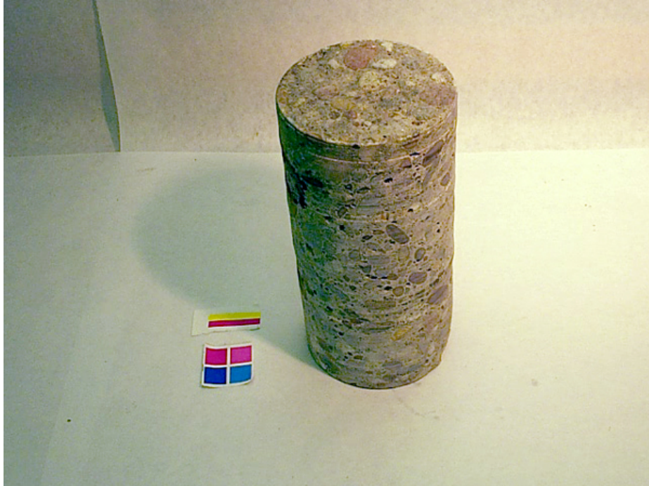
Figure 10: Core S-2, taken away from deteriorated area.
