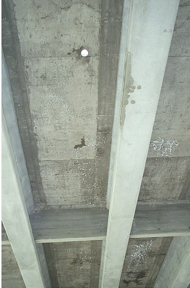
Figure 2: Beneath EB I-90 Tarkio interchange after coring.
