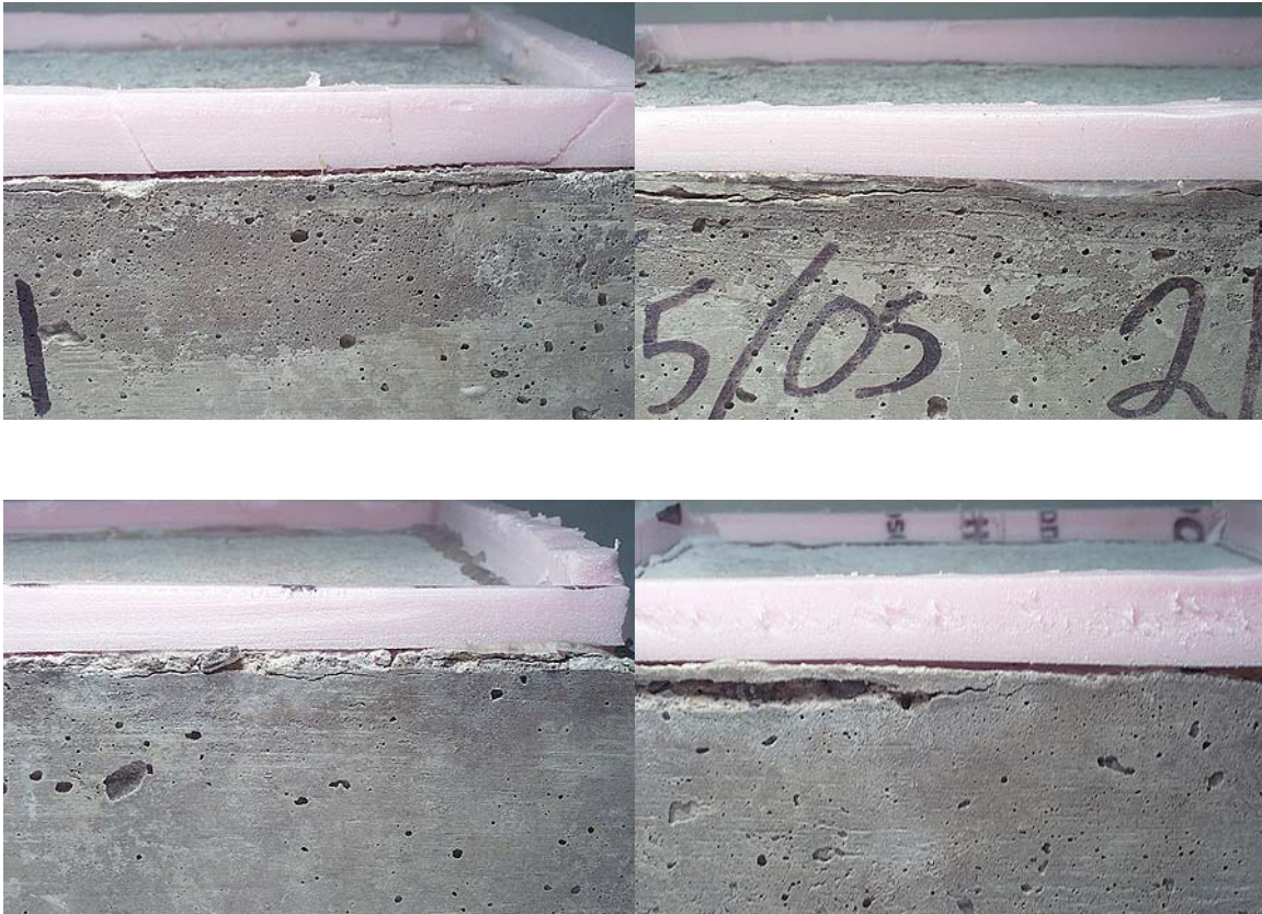
Figure 31: Cracks parallel to ponding surface along sides of prisms just below the pink edge dams typical of prisms exposed to \text{CaCl}_2 solution, and not observed on prisms exposed to other solutions.
