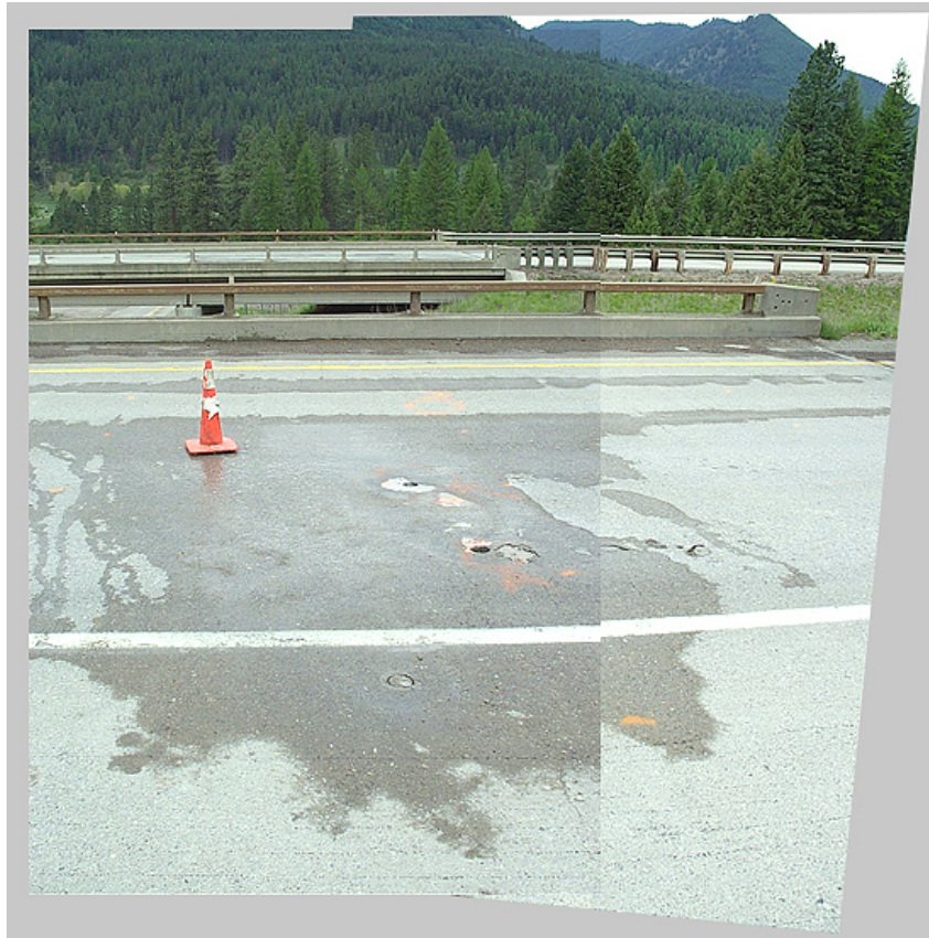
Figure 6: WB I-90 Sloway interchange bridge deck after coring.
