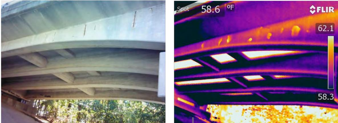
Figure 7: Standard and IR photos of bridge soffit delaminations (Mount Sterling, Kentucky)
