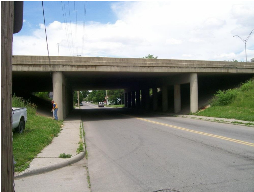
Figure 16. Slab bridge in Ohio where IR testing was conducted.
