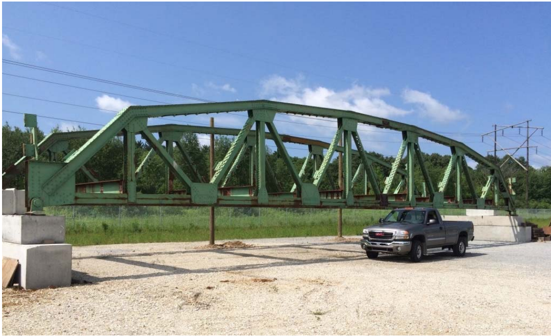
Erected 90 foot span pony truss
