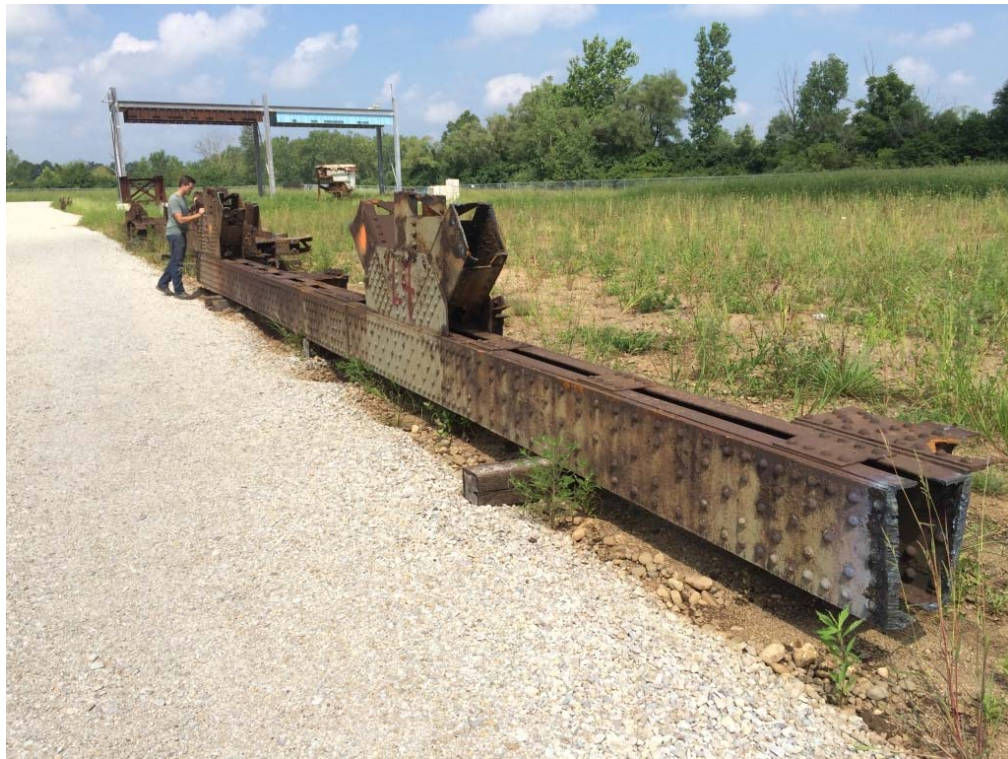
Chords from CSX RR bridge in Philadelphia
