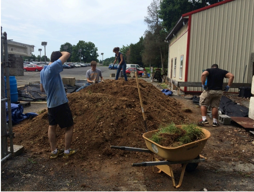
Figure 0.4. ALF Stockpile- Removing the organic soil from ALF soil.
