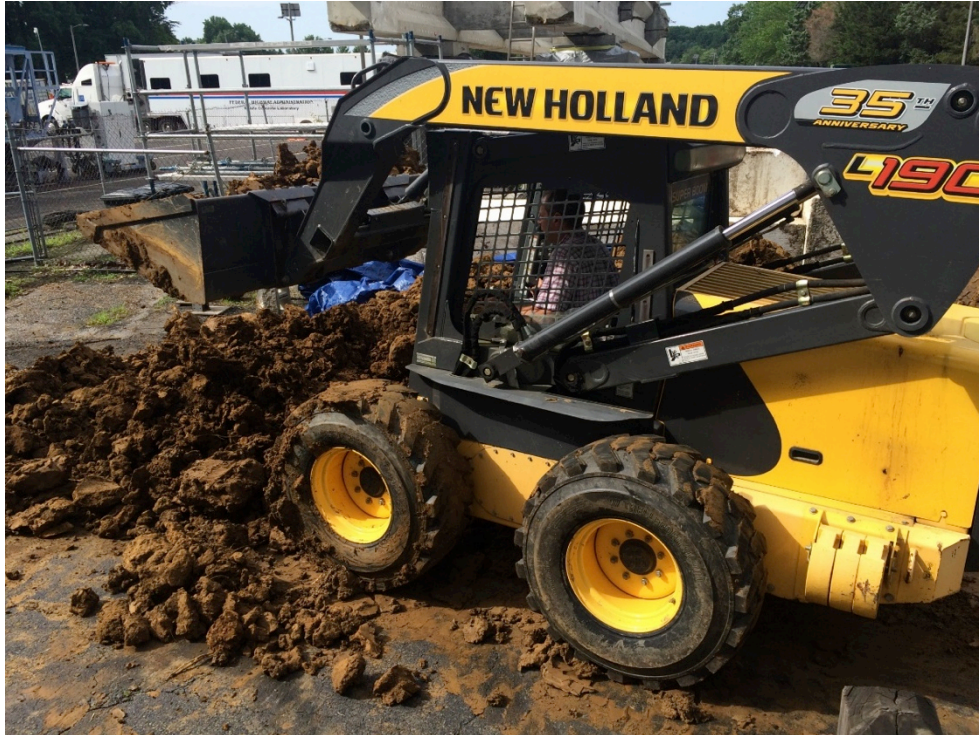
Figure 0.8. Use of skid-steer loader in breaking and spreading HPC for further drying.
