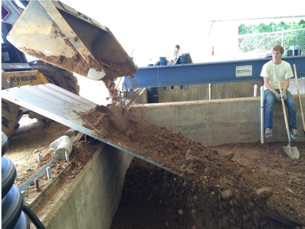
Figure 0.11. Use of ramp for transferring the material into the pits.
