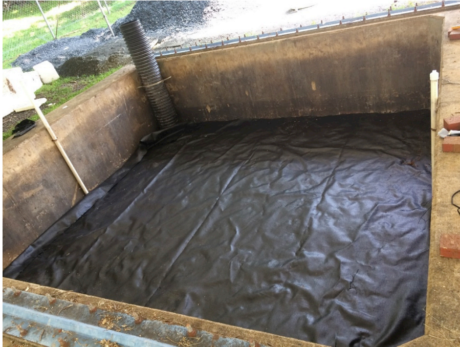
Figure 0.2. Placement of geotextile on top of the 1.2 m crushed stone.
