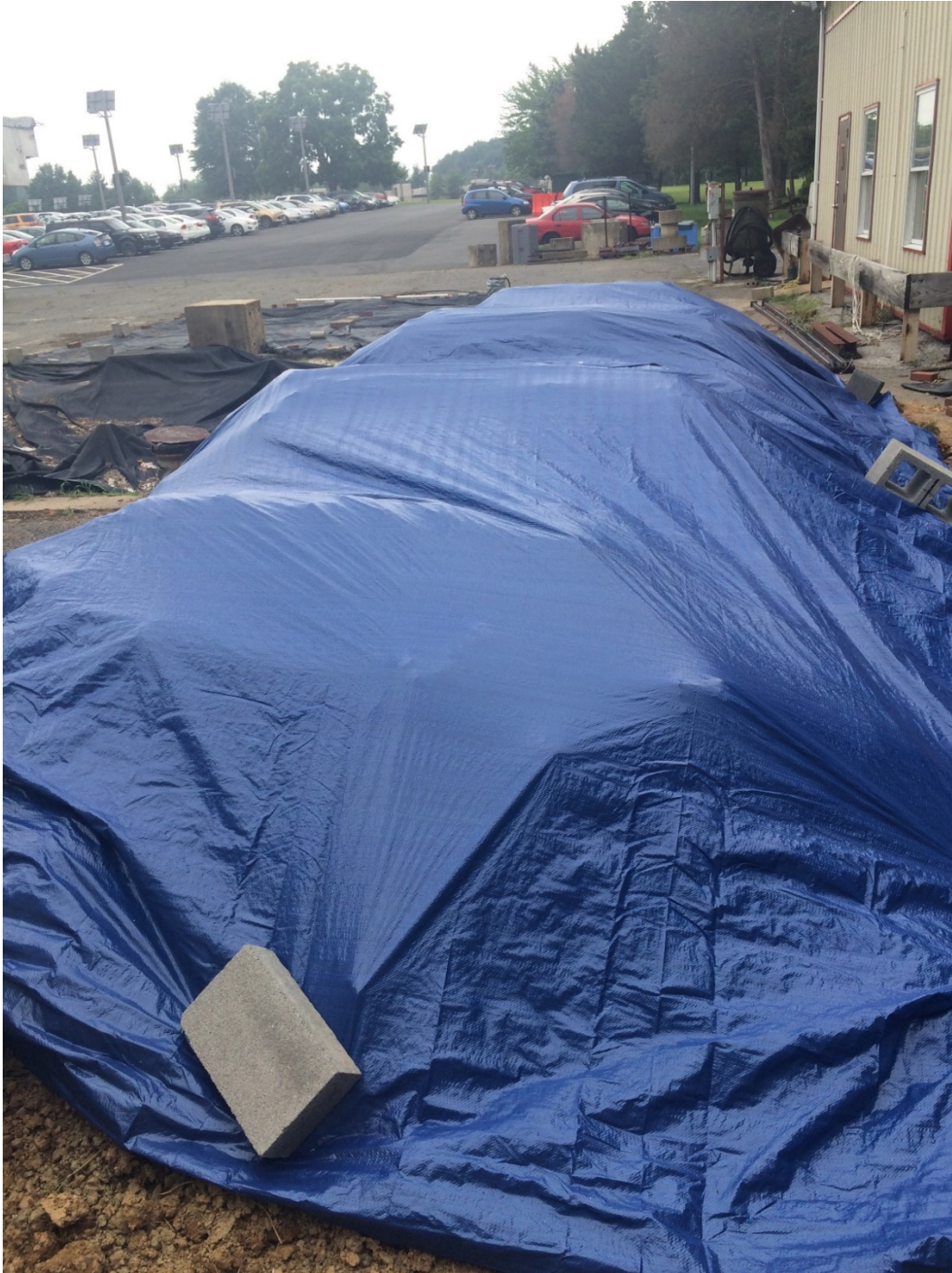
Figure 0.10. Covering the stockpiles.
