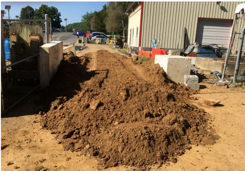
Figure 0.5. Spreading ALF stockpile for drying prior to compaction.
