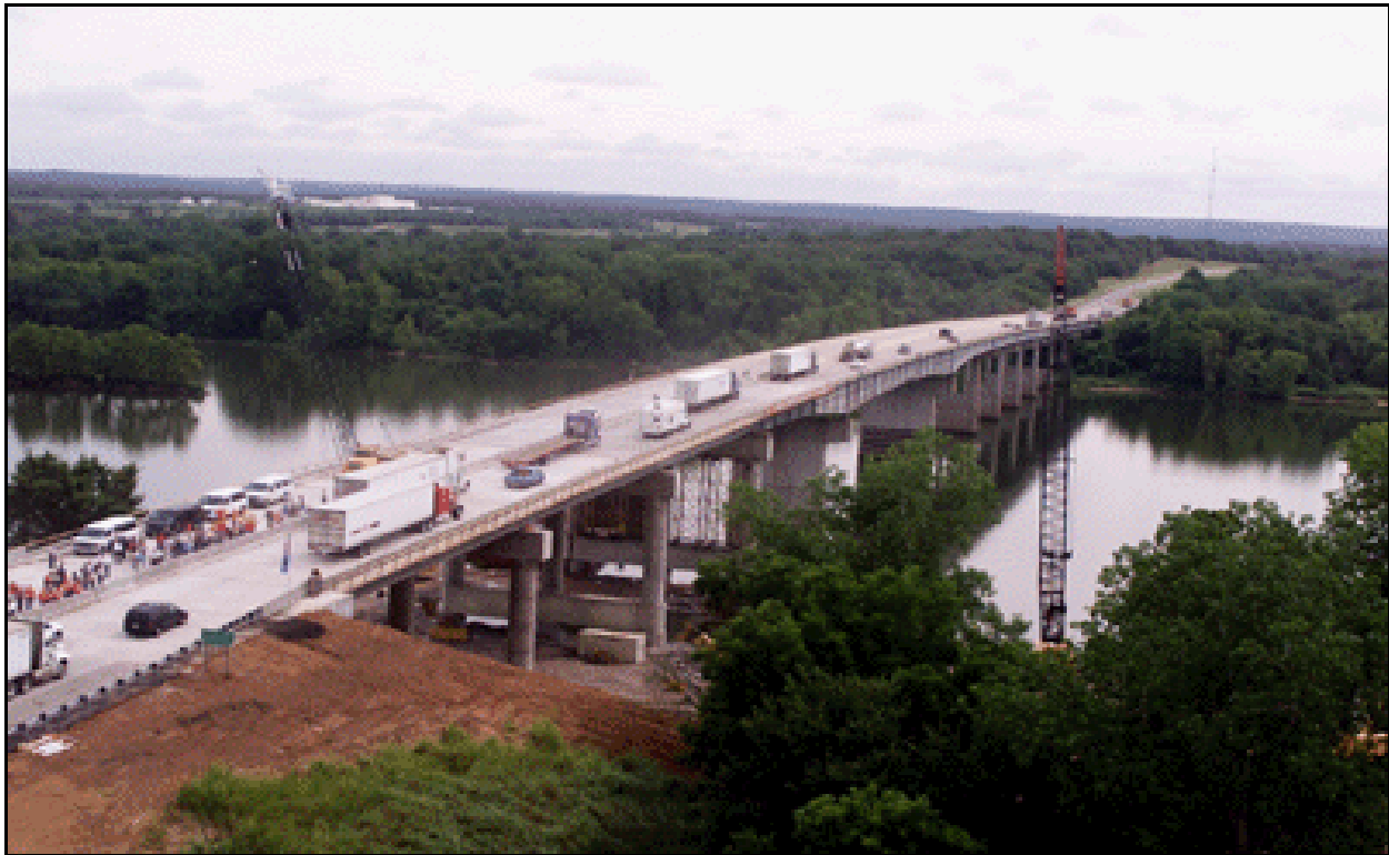
Figure 7 I-40 Bridge Re-Opened to the Traveling Public (Provided by ODOT)
