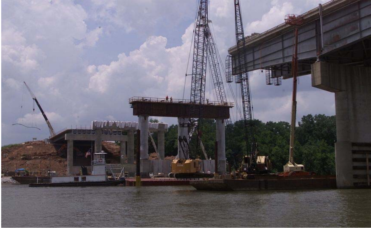
Figure 6 New Pier Structures (Provided by ODOT)
