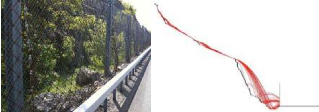
Figure 46. Comparison of an actual rockfall event (left) with the RocFall trajectory modeling results (right).
