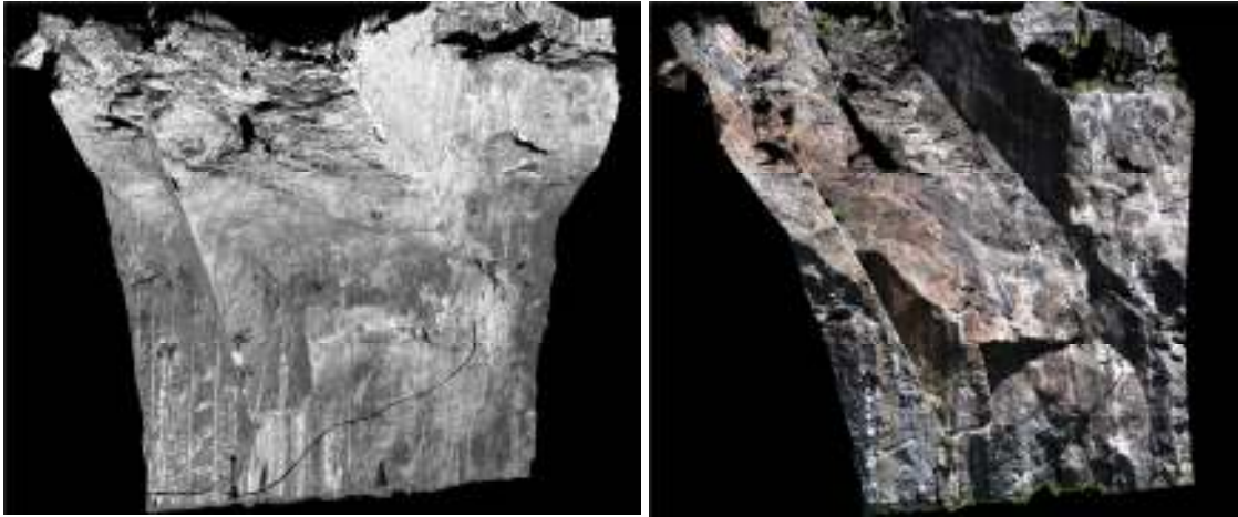
Figure 1. Scans from a highway rock slope in New Hampshire, from left, a) an intensity point cloud and b) a color point cloud.
