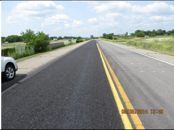
New 528' Coarse Chip Seal at MnROAD on Low Volume Road used for reference devices & inertial profiler evaluations
