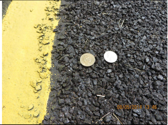
Close-up of new coarse chip seal on LVR
