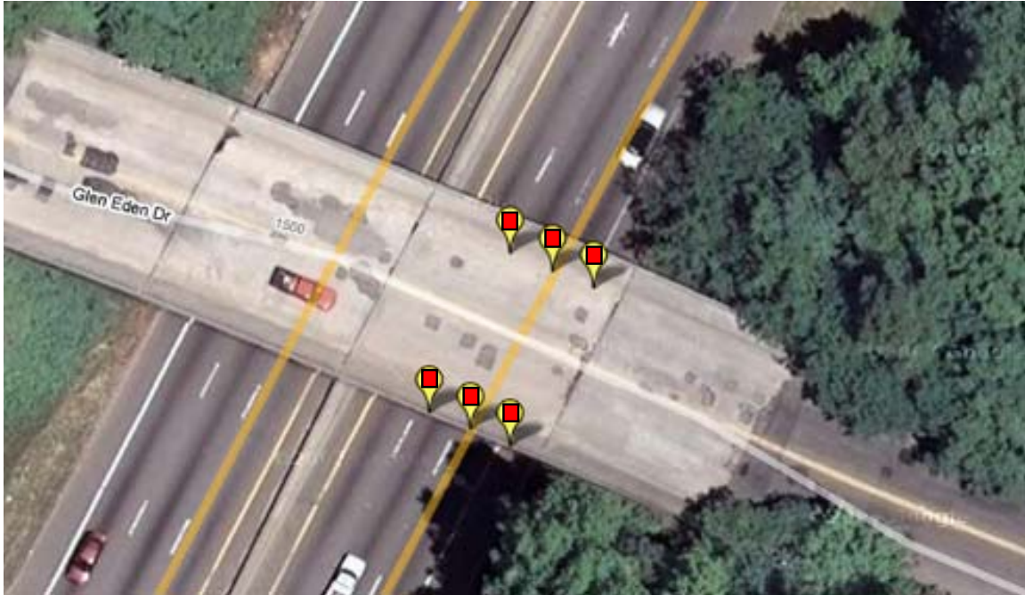
Figure 4.14. Terramatrix measurement locations for Glen Eden Drive bridge.
