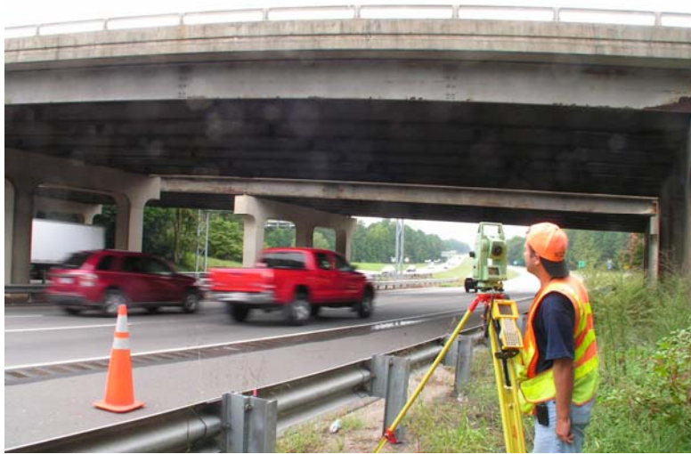
Figure 4.11. NCDOT special survey of vertical clearance at selected bridges.
