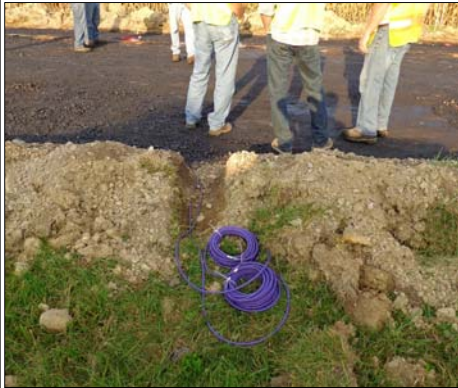
Pressure cells on top of subgrade
