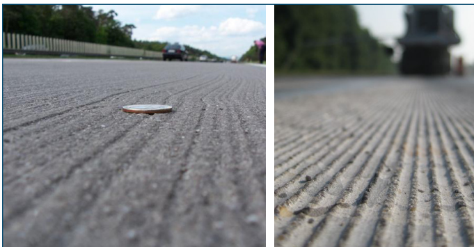
Figure 6. Drag textured and diamond ground concrete pavements
