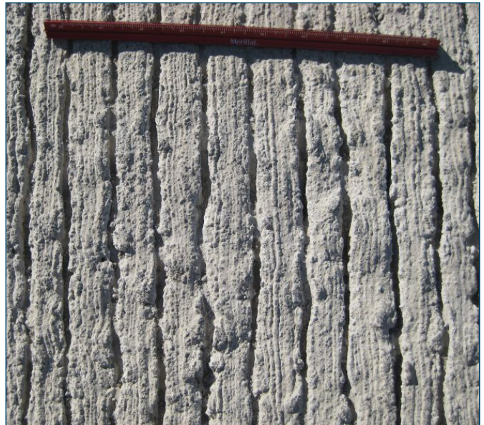
Figure 15. Excessive intermediate aggregates in close proximity to the surface leading to undesirable texture
