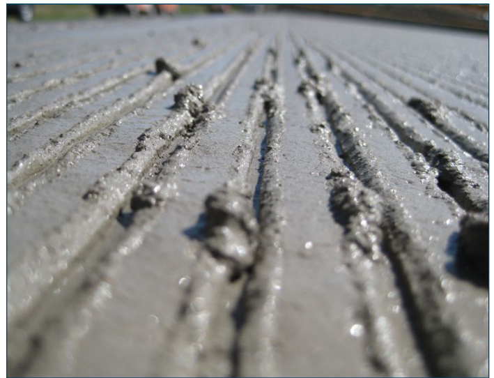
Figure 19. Redeeposited mortar on the surface of the lands between the tined grooves
