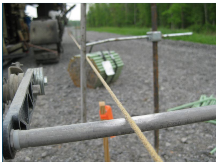
Figure 37. Sensor rods that track alignment and elevation
