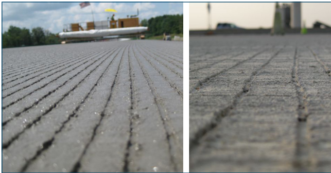
Figure 5. Longitudinal and transverse tined concrete pavements
