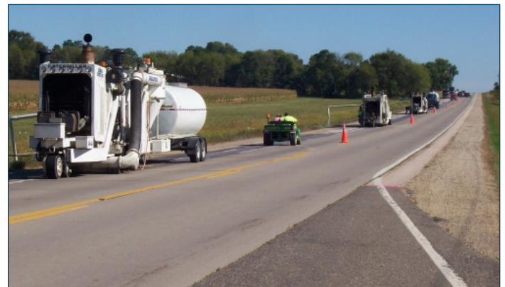
Figure 59. A grinding large-scale concrete pavement resurfacing operation
