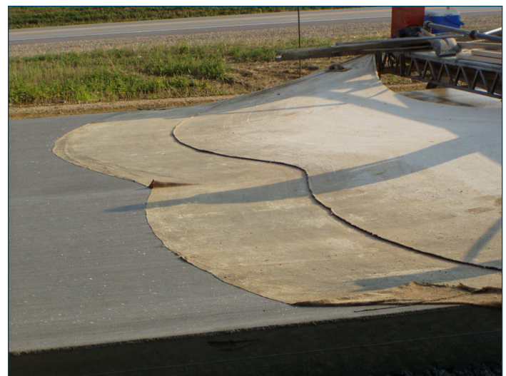
Figure 54. Burlap drag attached to a work bridge
