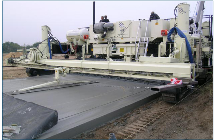
Figure 44. Automatic longitudinal float attached to the back of a paver
