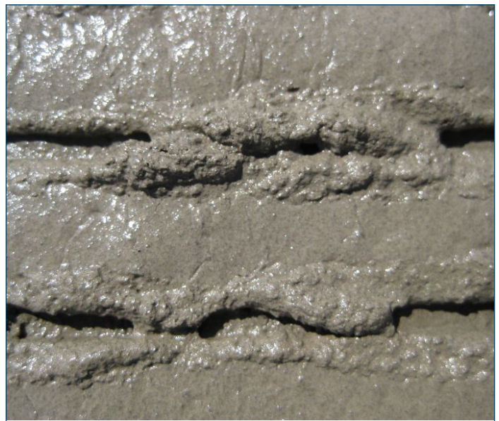
Figure 16. Excessively fluid mortar leading to closing of tined grooves
