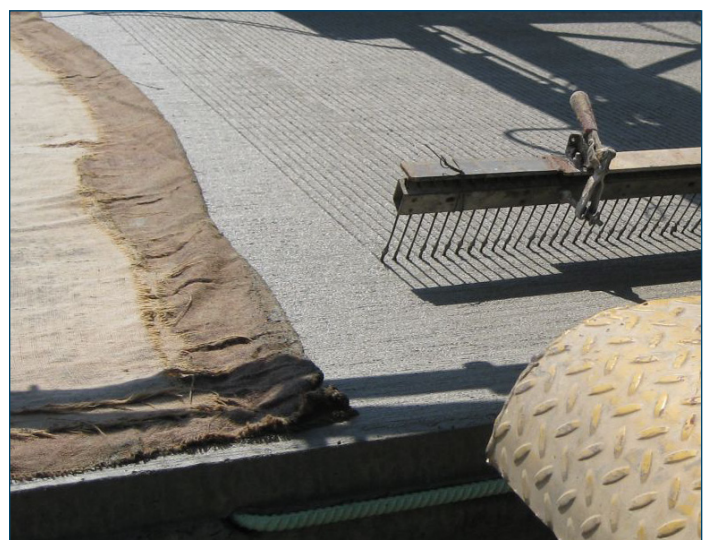
Figure 20. Drag pretexture applied prior to tining operations
