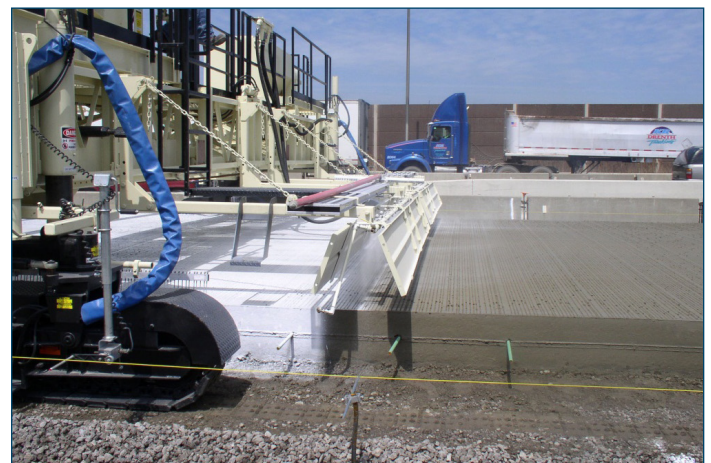
Figure 57. Illustration of curing equipment on texture-cure machine following good practice
