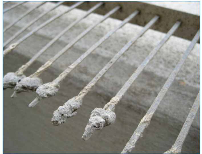
Figure 22. Excessive buildup of hardened mortar on tines
