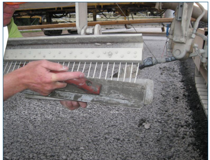
Figure 23. Simple technique to clean hardened mortar from tines
