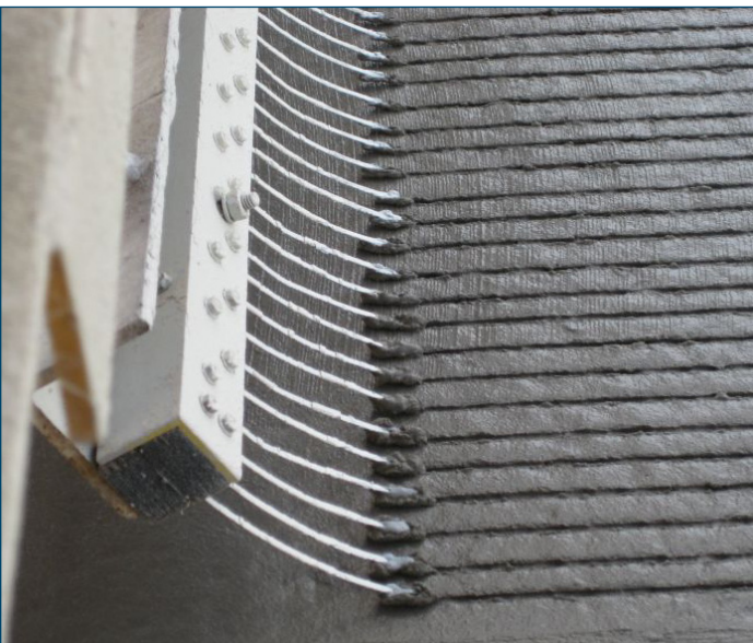
Figure 25. Angle of tines affecting contact with concrete surface
