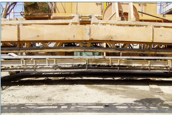
Figure 43. Forming pan set for a crowned pavement
