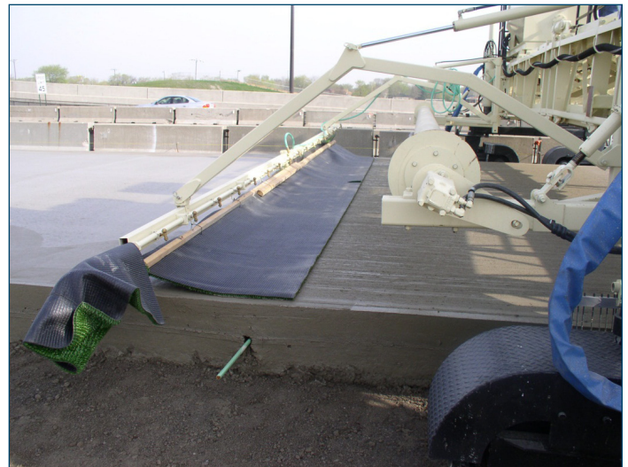
Figure 53. Turf drag attachment on a texture machine
