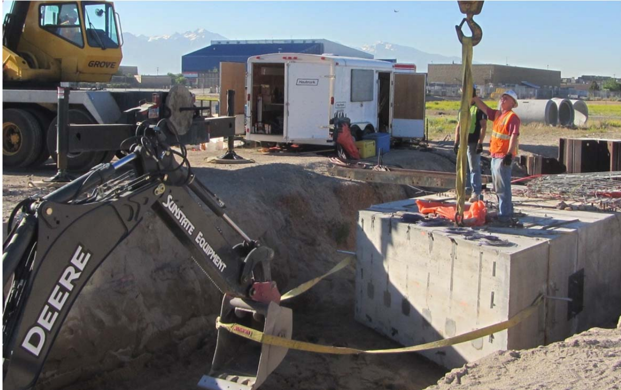
Figure 3.12: Removal of the 30° Concrete Wedge
