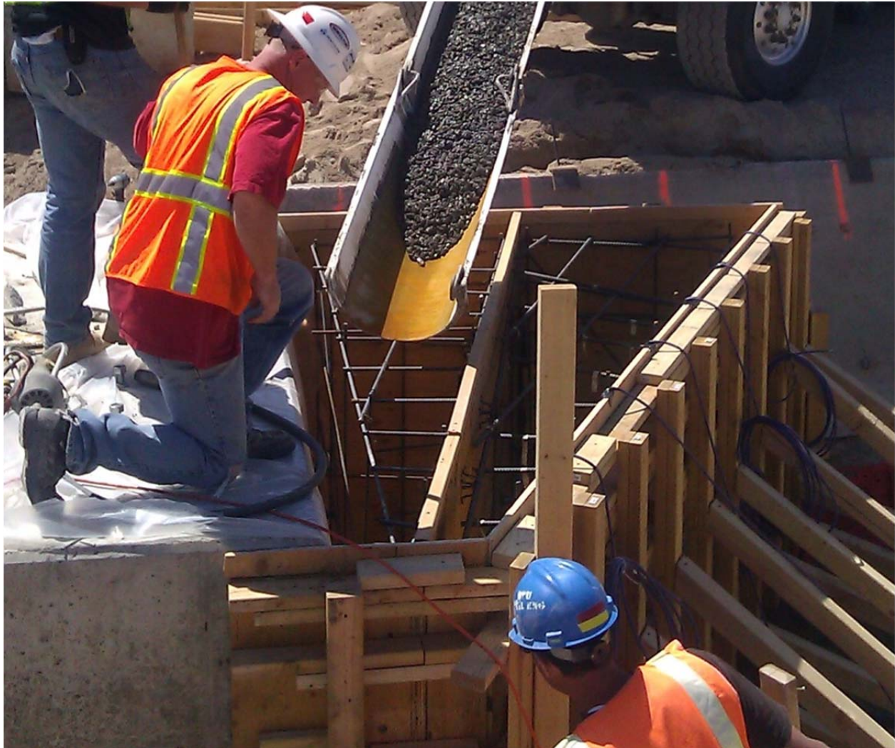
Figure 3.6: Simultaneous Casing of the 15° and 30° Wedges
