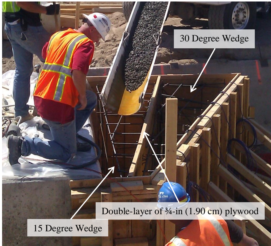
Figure 3-4: Simultaneous casting of 15° and 30° wedges
