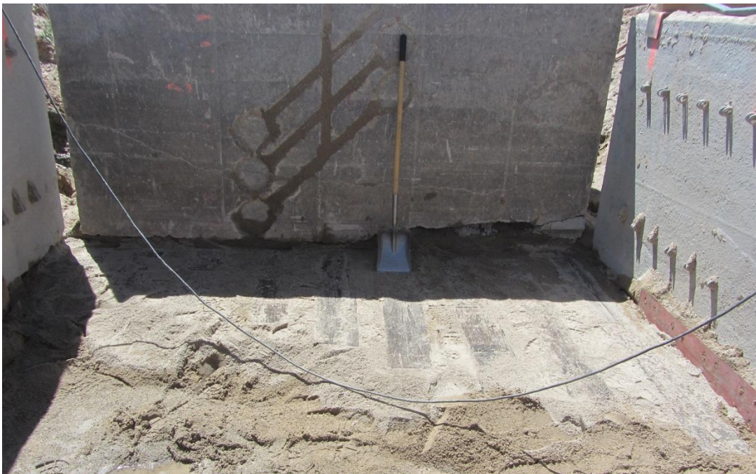
Figure 3-10: Railroad tie foundation for 15° and 30° wedges with sand compacted between ties
