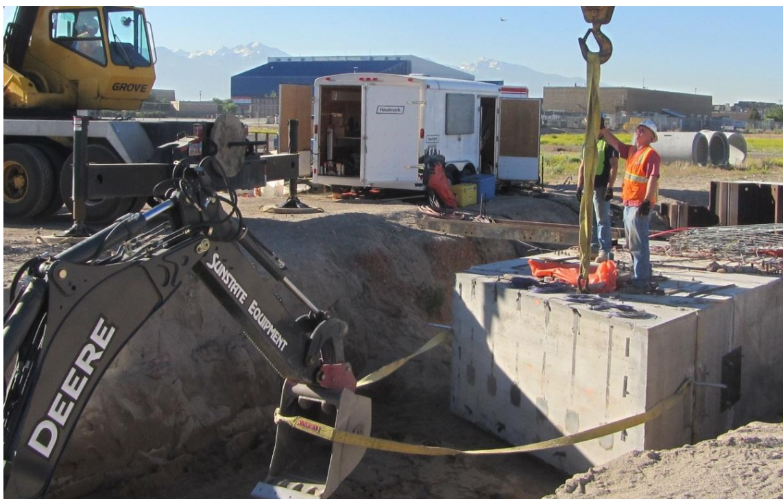
Figure 3-12: Removal of 30° wedge
