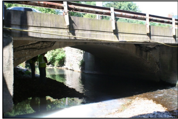
Figure 2-5 - Michigan Avenue Bridge
