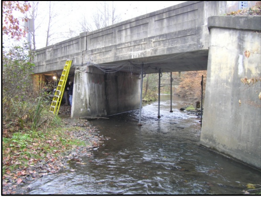
Figure 2-2 - Tams Slab Bridge
