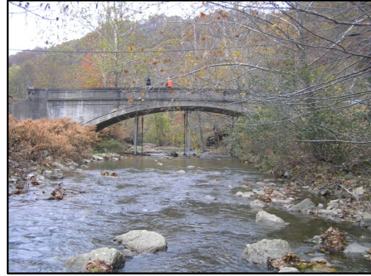
Figure 2-3 - Amigo Arch Bridge
