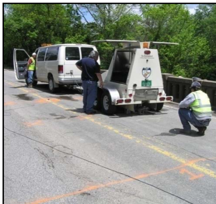
Figure 2-9 – FWD on the Bridge for Testing
