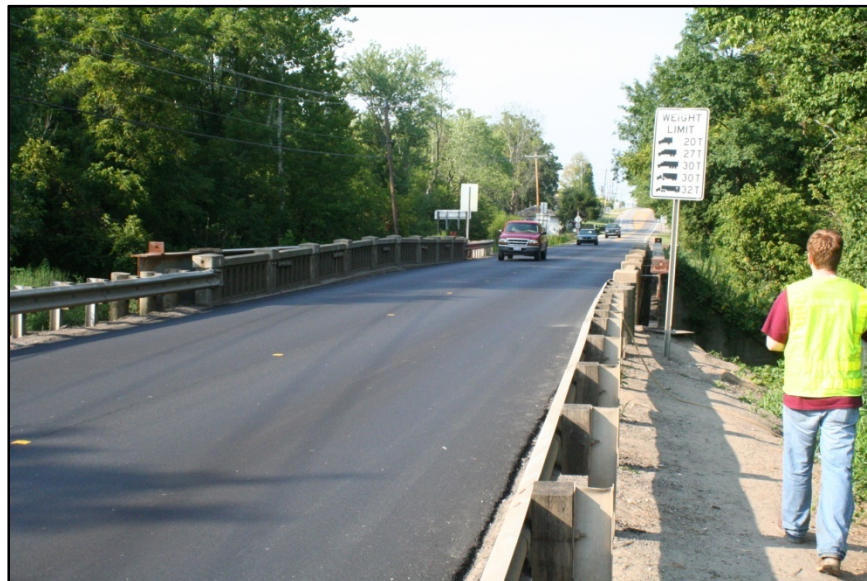
Figure 2-1 - Barnett Bridge (Posting was Removed)
