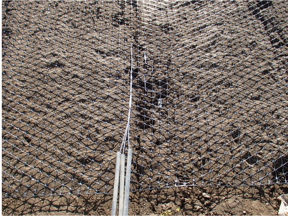
Figure 32: Typical lead wire installation with protective tubing.
