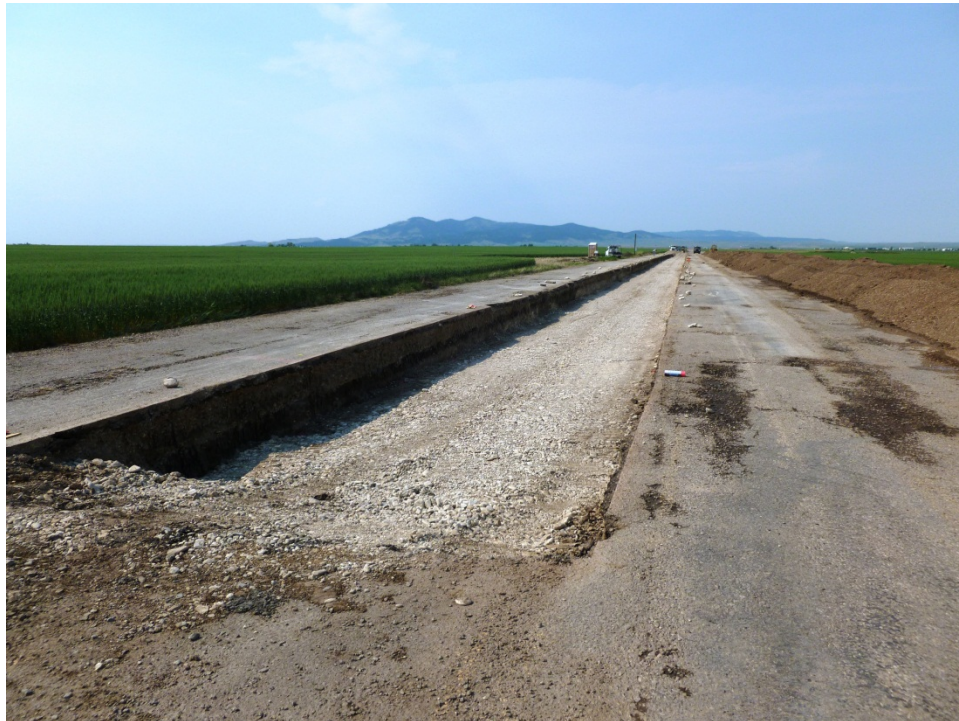
Figure 9: Completed trench.
