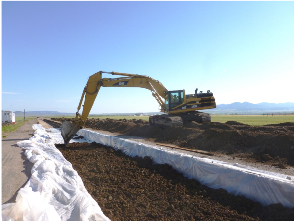
Figure 10: Filling lined trench with subgrade.
