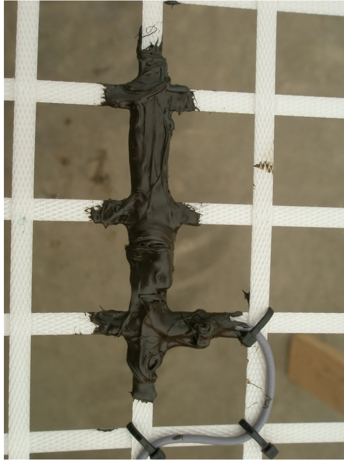
Figure 35: Completed strain gage installation with protective coating.
