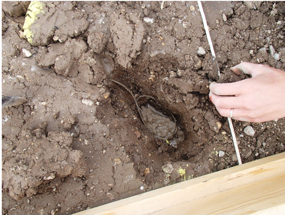
Figure 38: Installation of pore water pressure sensor in subgrade.
