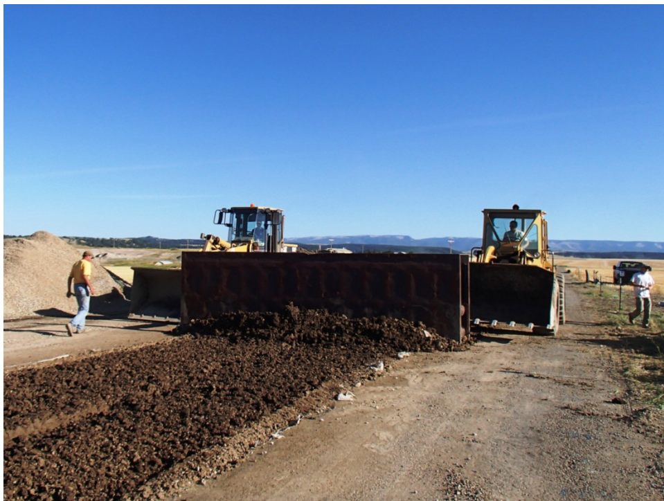
Figure 14: Screeding final subgrade layer.
