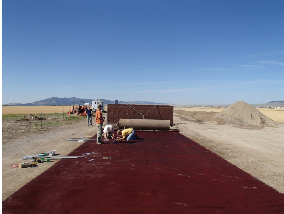
Figure 21: Installed geosynthetic.
