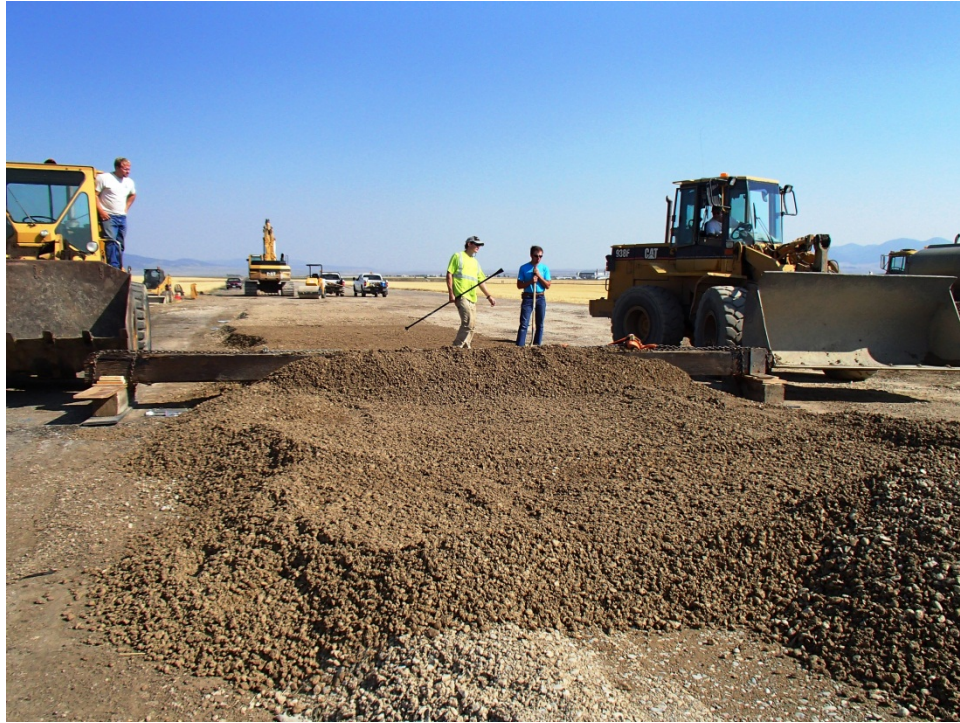
Figure 22: Screeding gravel surface.
