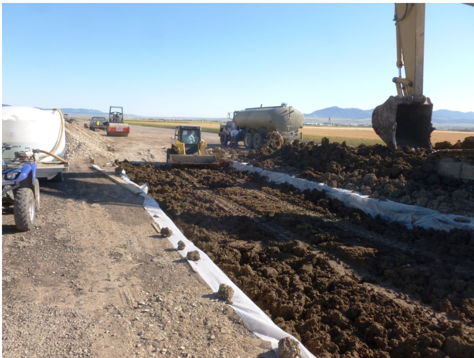
Figure 12: Tracking freshly placed subgrade with track-mounted skid-steer.
