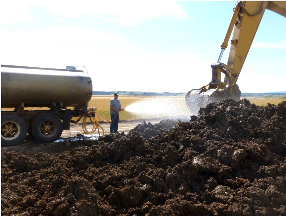
Figure 11: Watering and mixing subgrade with excavator.
