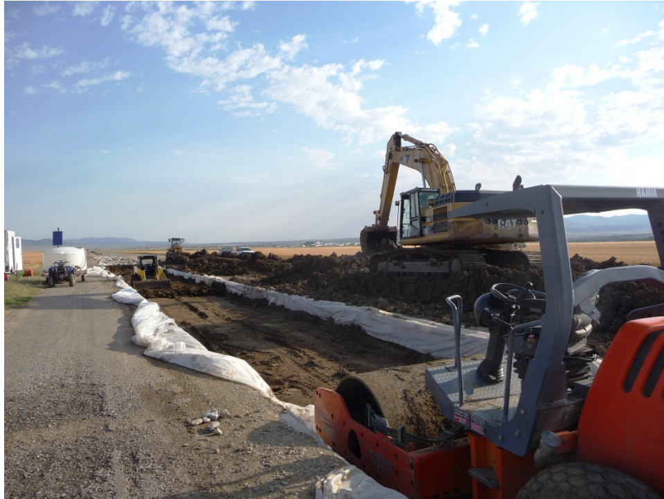
Figure 13: Smooth-drum roller used to compact subgrade.
