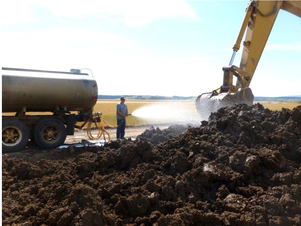
Figure 1: Watering and mixing subgrade with excavator.
