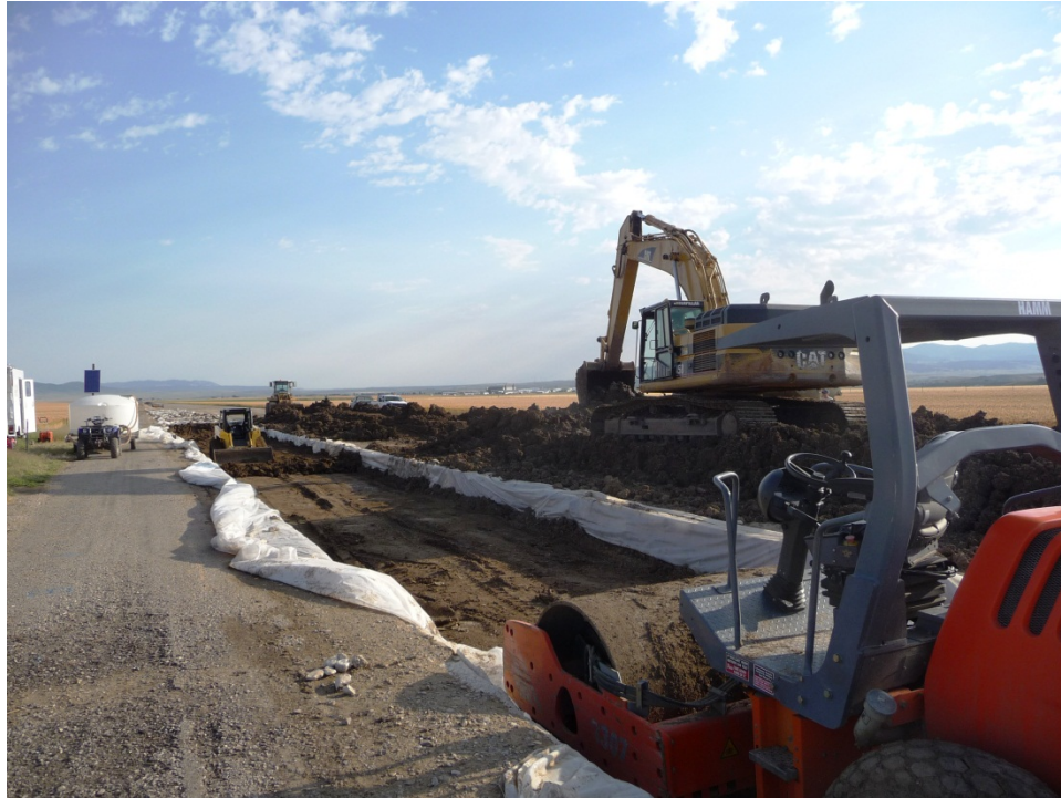
Figure 3: Smooth-drum roller used to compact subgrade.
