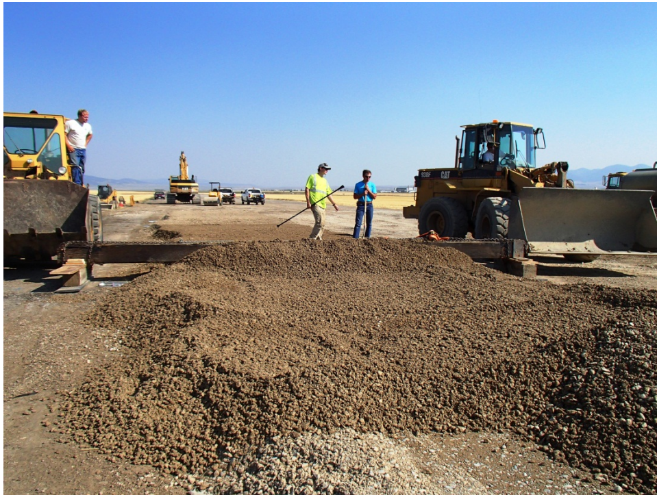
Figure 6: Screeding gravel surface.
