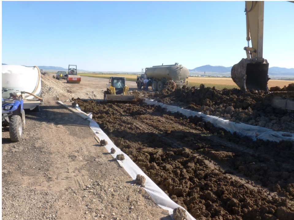
Figure 2: Tracking freshly placed subgrade with track-mounted skid-steer.
