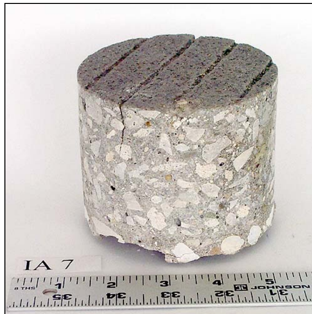
Figure 3.7. Core as received from Iowa site, with surface crack, (IA_07).
