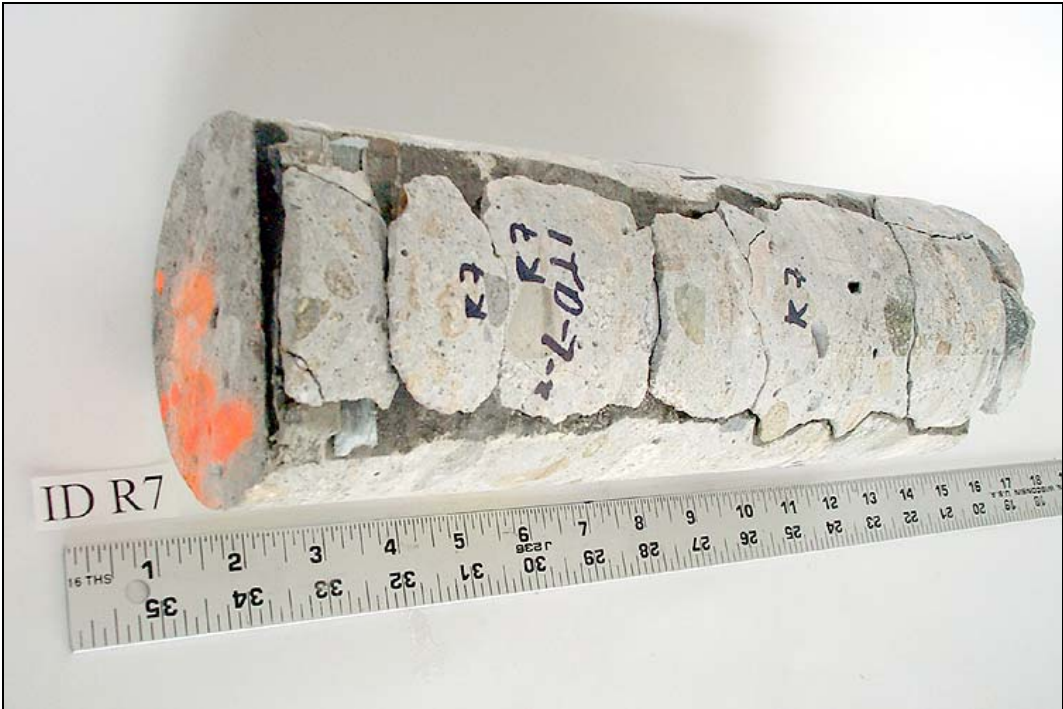
Figure 3.3. Core as received from Idaho site, right-most lane, at joint, (ID_R07).
