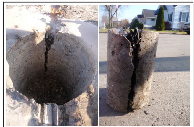
Figure 26. Coring at deteriorated joints to help identify causes of failure
