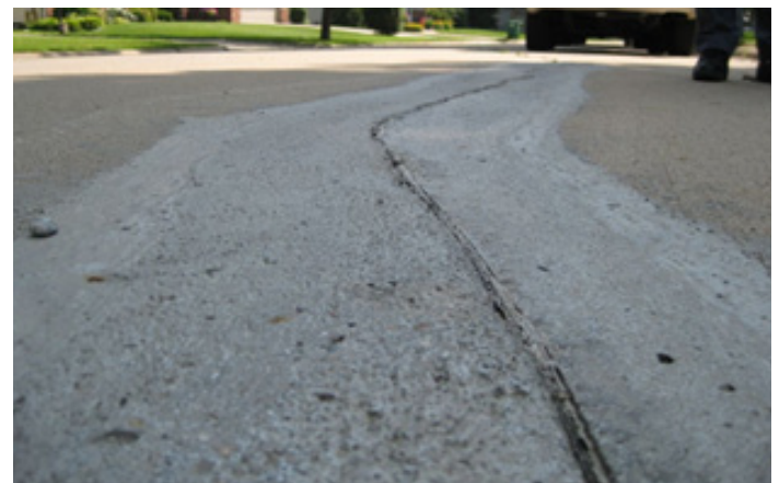
Figure 39. Completed patch (Source: The Transtec Group)
