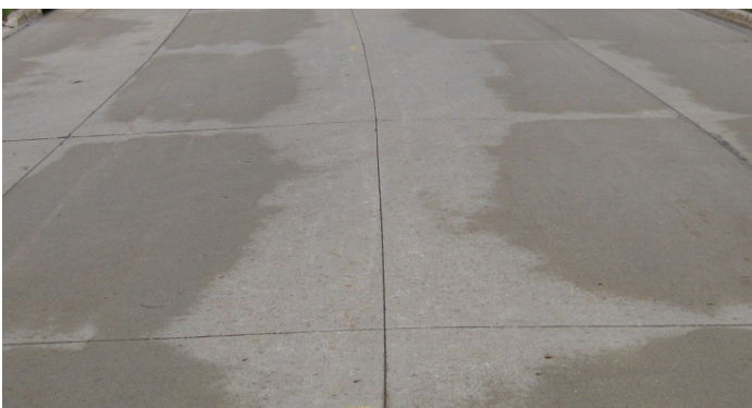
Figure 36. Example of effective drainage of unsealed joints
