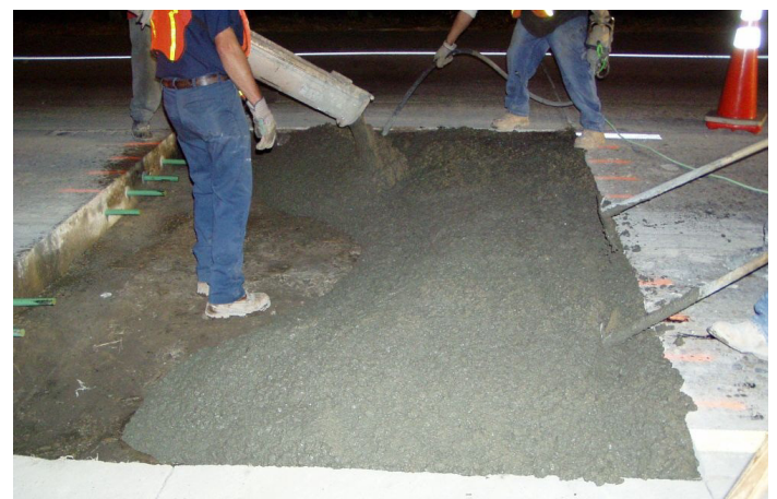
Figure 40. Full-depth patching
