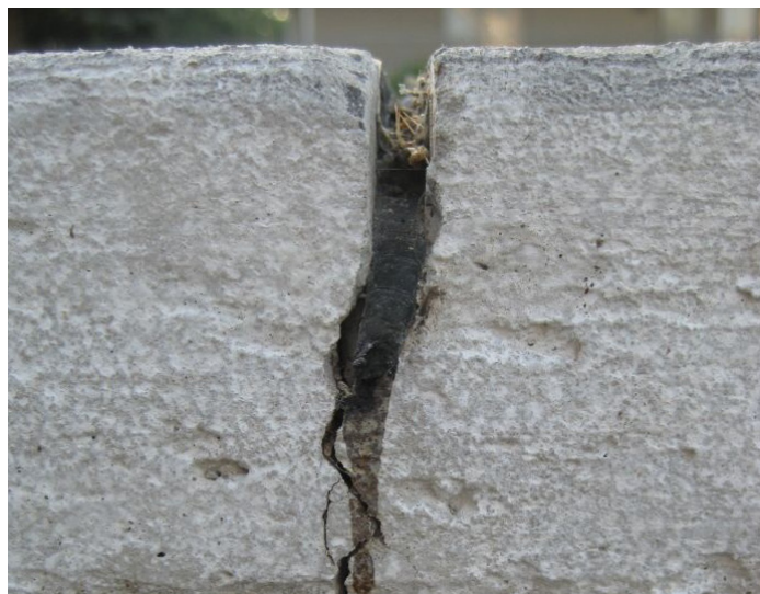
Figure 32. Joint filled with hot-pour sealant (Source: The Transtec Group)
