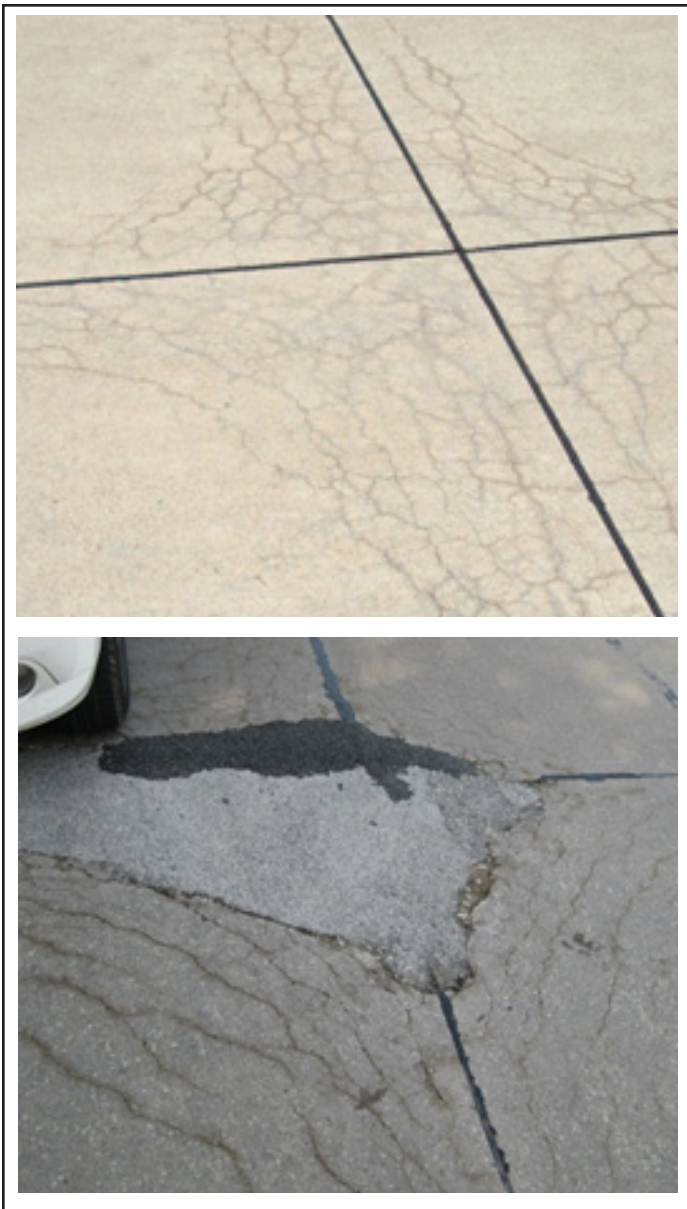
Figure 16. D cracking of low severity (top) and high severity (bottom) (Source: The Transtec Group)
