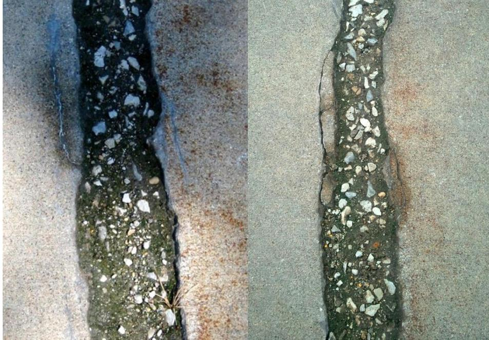
**Figure 4. Sample of damage increasing over time (July 2011 to July 2012)**
