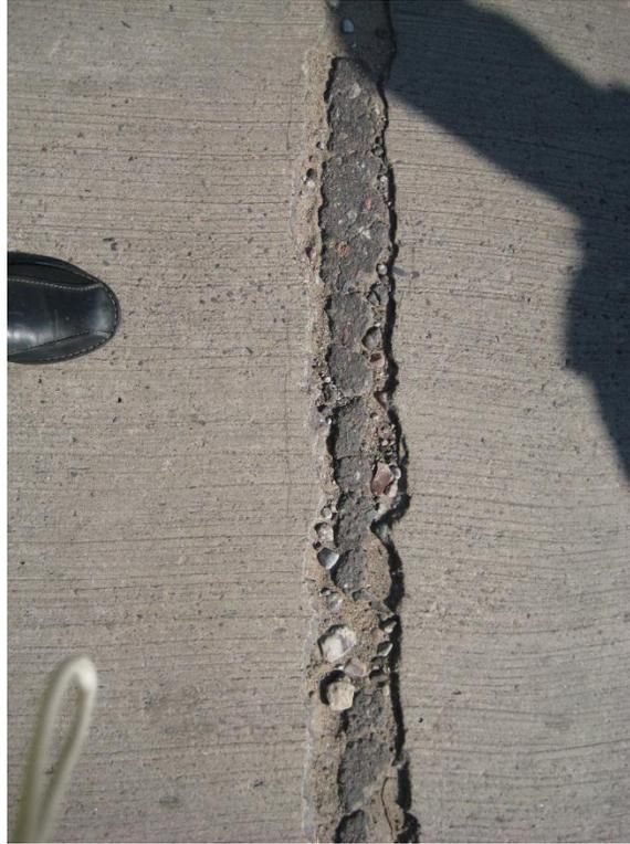
**Figure 2. Distress in transverse joint**
