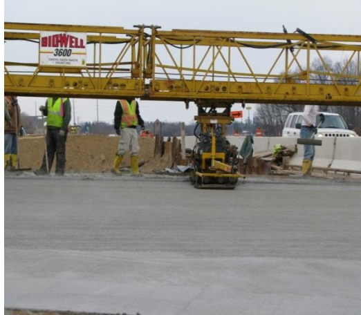
Figure 9. Concrete being finished
