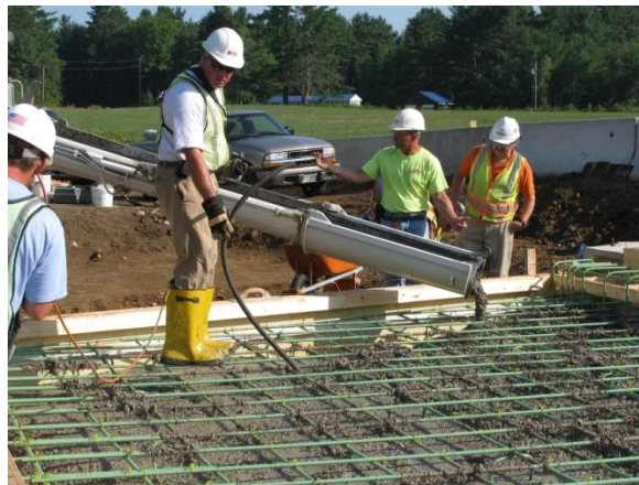
Figure 8. Concrete being vibrated
