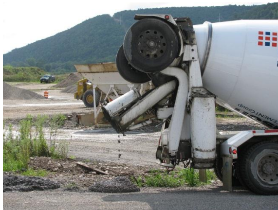
Figure 5. Concrete being discharged
