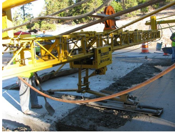
Figure 11. Concrete surface being sealed by Auto-Float
