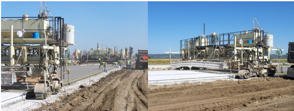
Figures 10 and 11. Concrete being finished and curing compound being applied
