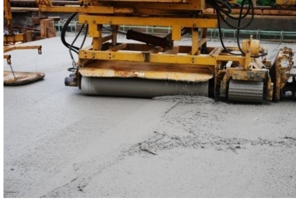
Figure 10. Concrete being finished
