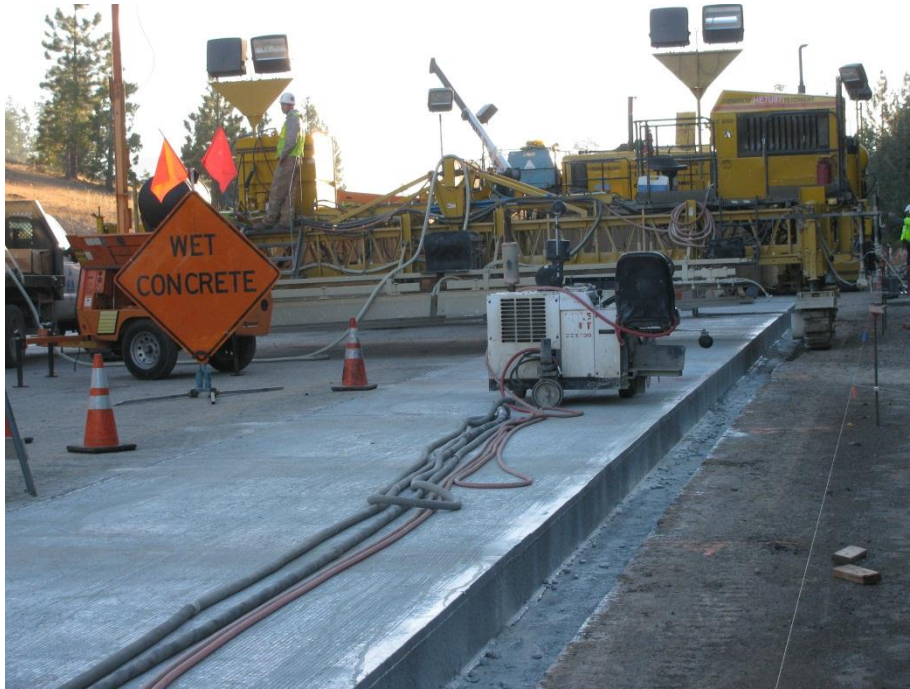
Figure 1. I-80 rigid pavement reconstruction, Emigrant Gap, California
