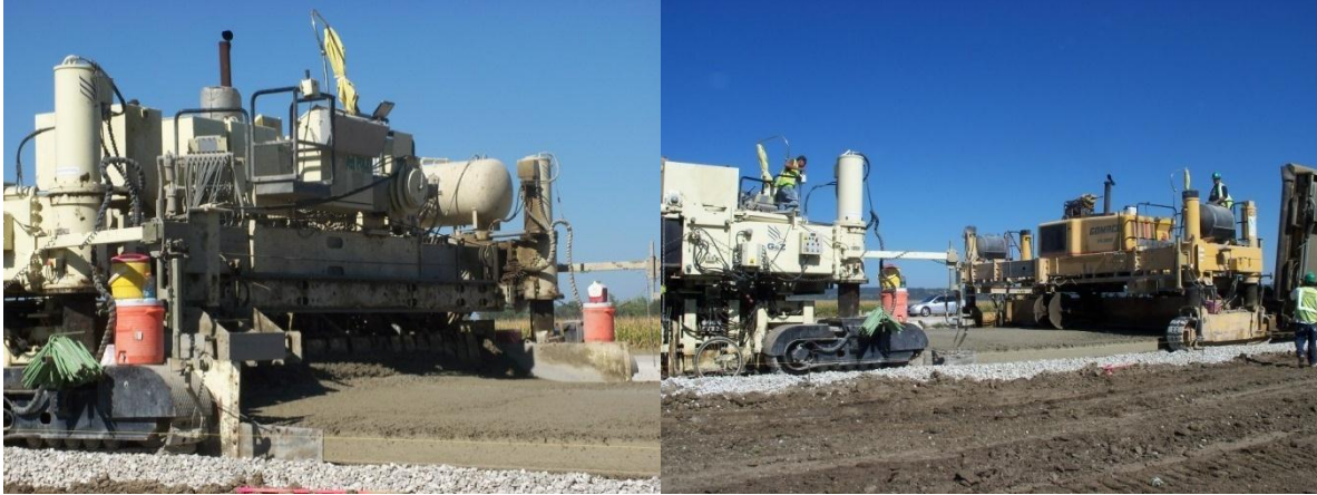
Figures 8 and 9. Concrete passing through the paver
