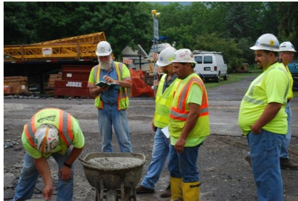
Figure 6. Concrete being tested by PennDOT technicians
