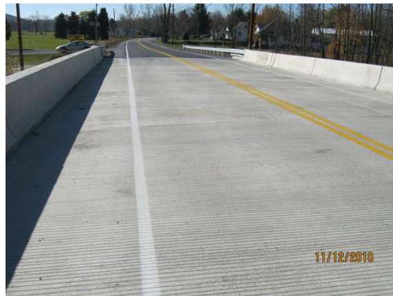
Figure 14. Bridge deck surface four months after construction
