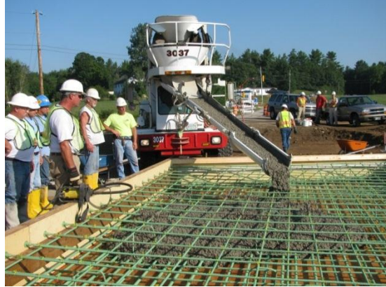
Figure 7. Bridge deck with concrete being placed
