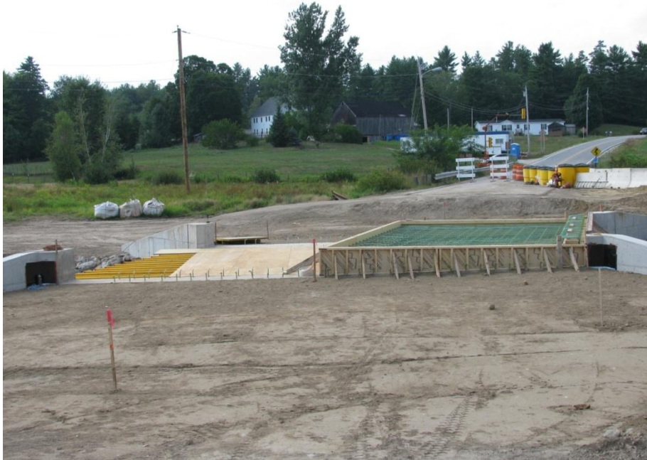
Figure 1. Route 107 bridge deck in Epsom, New Hampshire
