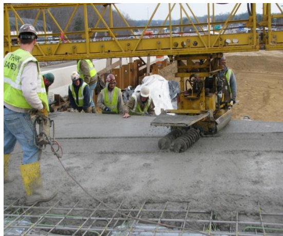
Figure 8. Concrete being placed
