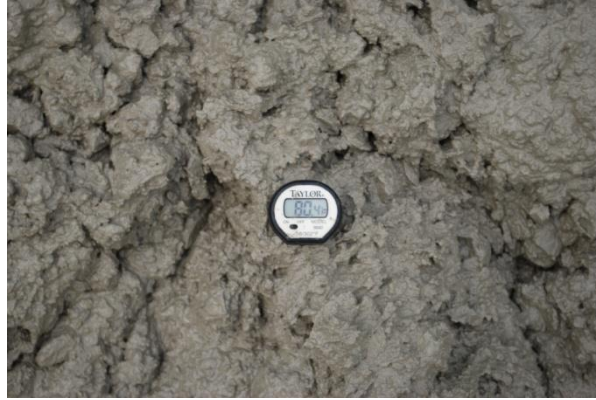
Figure 13. Concrete temperature being tested by sensor
