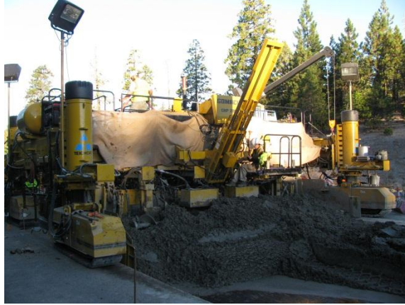
Figure 8. Concrete passing through the paver
