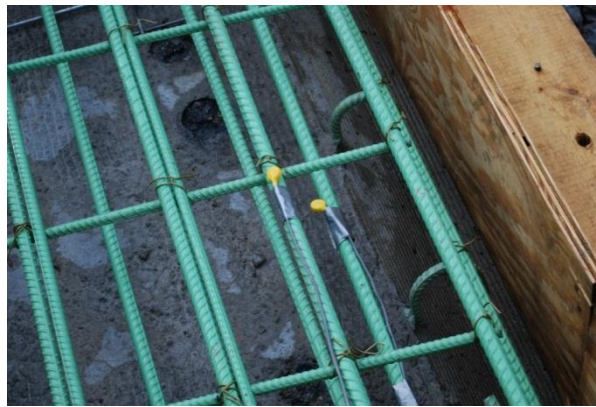
Figure 11. Two i-buttons being embedded on site
