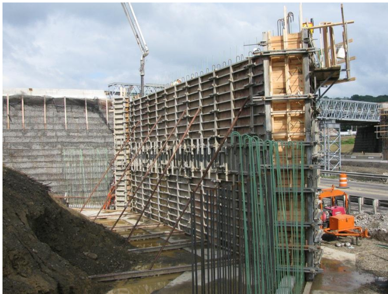
Figure 7. Concrete being placed in the abutment stem structure
