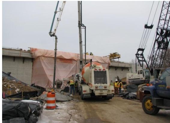
Figure 10. Concrete heated tent enclosure below the deck
