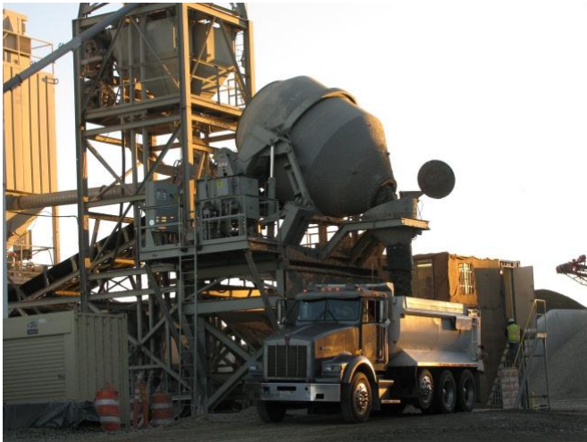
Figure 6. Concrete being discharged at central mix plant
