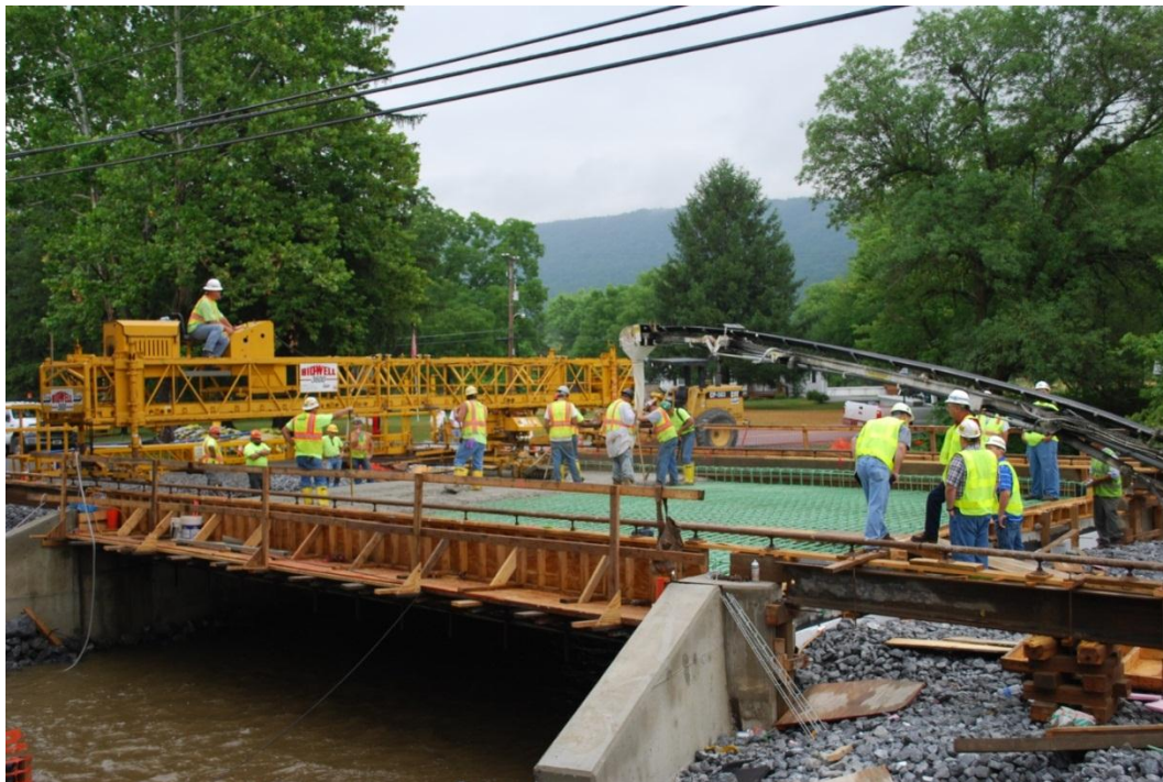
Figure 1. State Route 36 Section 20 bridge deck
