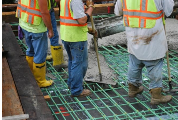
Figure 7. Concrete being spread by construction crews
