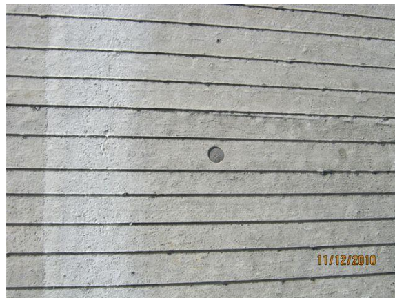
Figure 15. Bridge deck surface four months after construction
