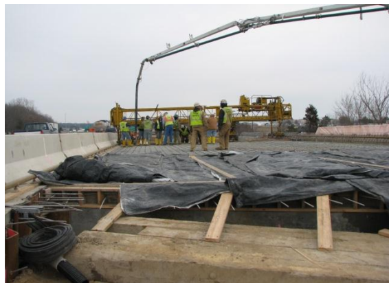
Figure 11. Curing blankets for concrete curing
