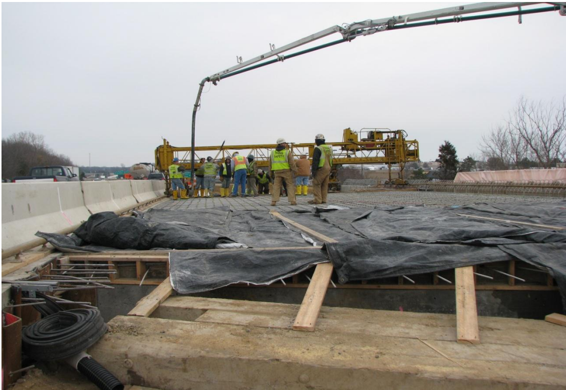
Figure 1. I-94 Riverside drive bridge deck placement
