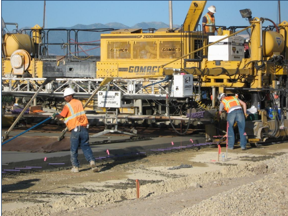
Figure 3. Paving operation at 10400 South, Salt Lake City, Utah
