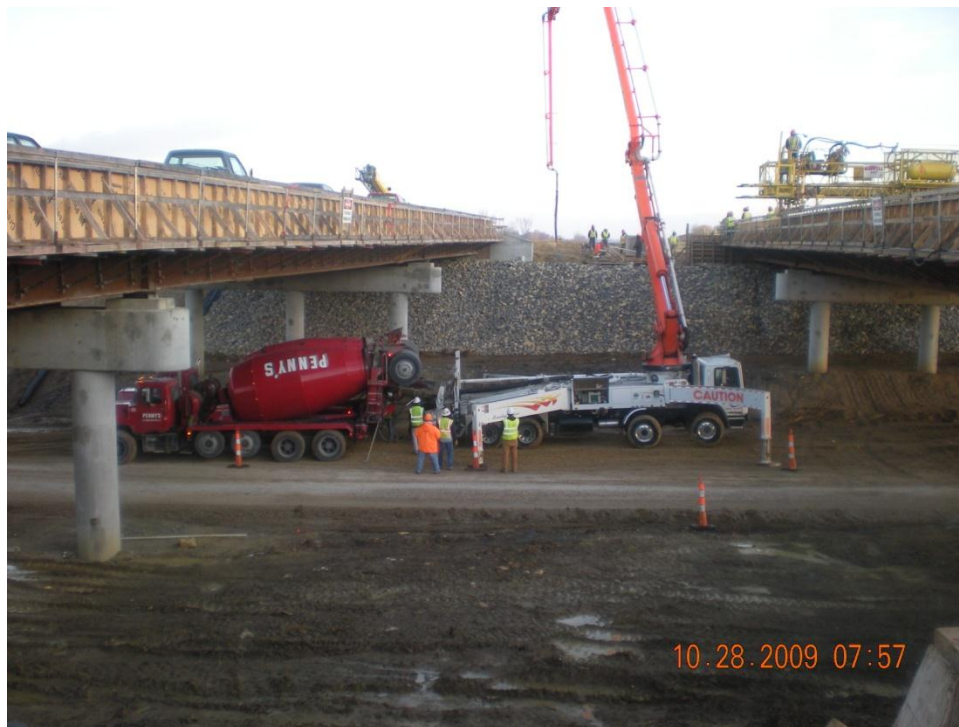
Figure 1. US 59 bridges (southbound-left and northbound-right)
