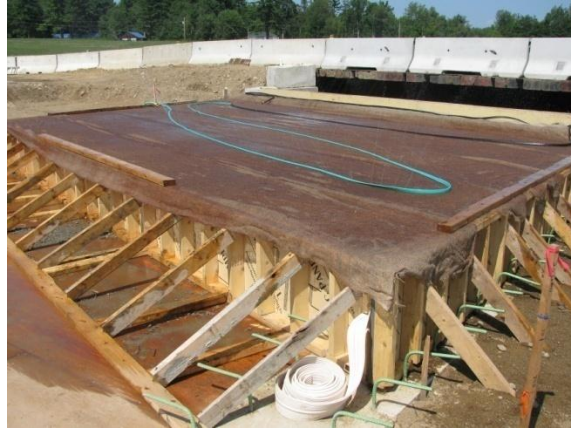
Figure 13. Concrete being cured with burlap
