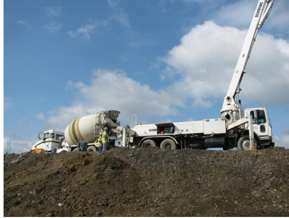
Figure 6. Concrete being pumped
