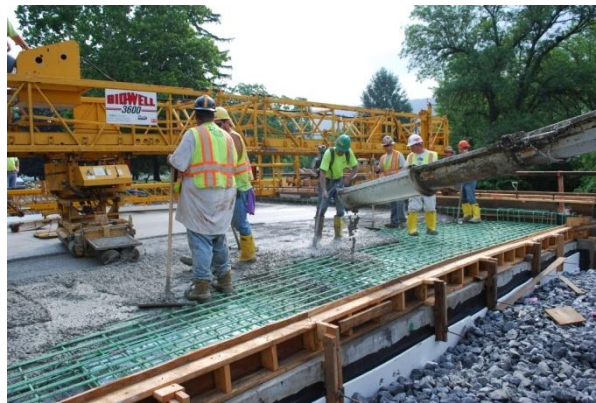
Figure 12. Concrete being vibrated
