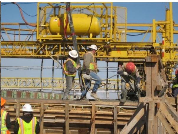
Figure 7. Construction crew placing concrete, pouring and vibrating
