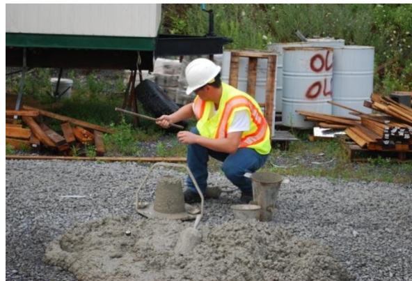
Figure 8. Concrete being tested by National CP Tech technician
