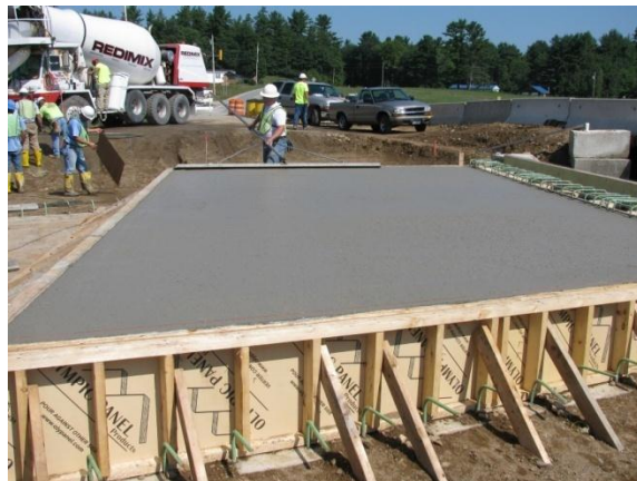
Figure 12. Concrete being finished
