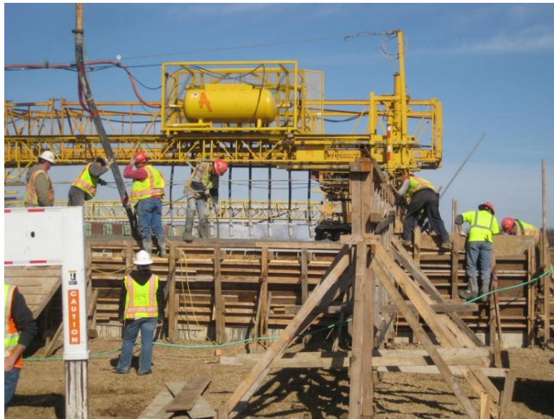
Figure 10. Concrete being placed and vibrated
