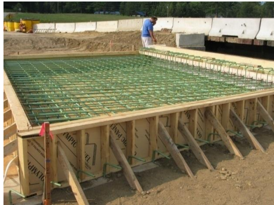
Figure 6. Bridge deck with removable wood form
