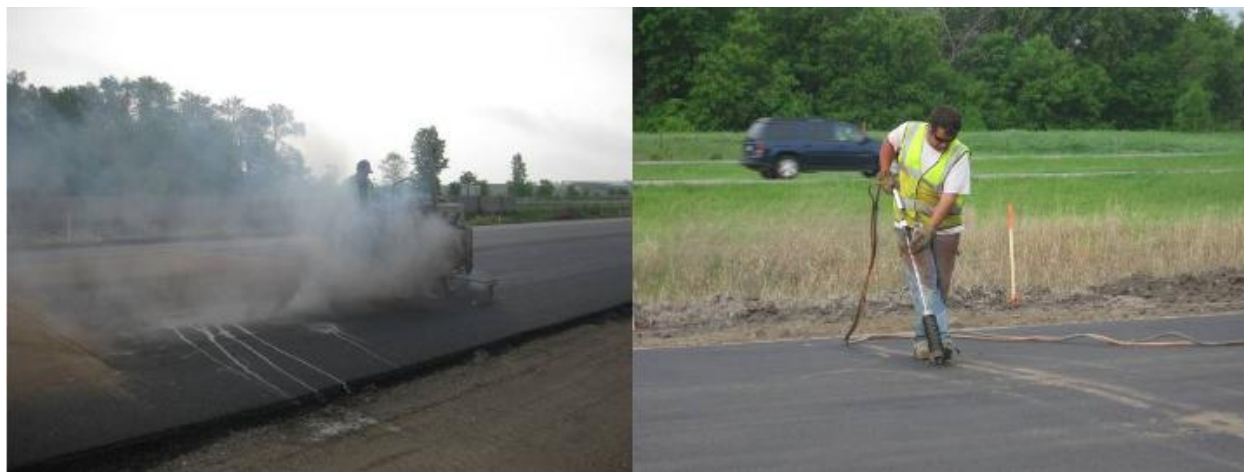
Figure 5-15. Sawing joints in the AC layer which correspond to the joints in the underlying PCC layer (left) and sealing the newly sawn joints (from Rao et al 2011)
