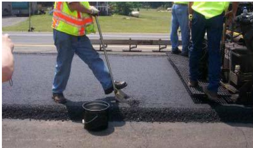
Figure 5-20 Shoveling material from above plates
