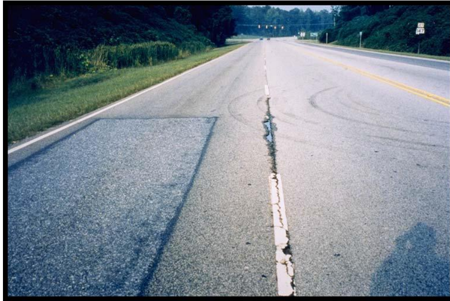
Figure 5-11: Raveled longitudinal joint (Brown, 2006)
