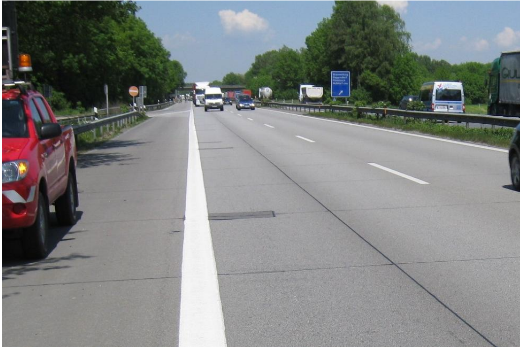
Figure 5-112 SMA over PCC along A93 in Germany, rectangular patch repair visible next to red traffic diversion truck (Rao SHRP 2010)
