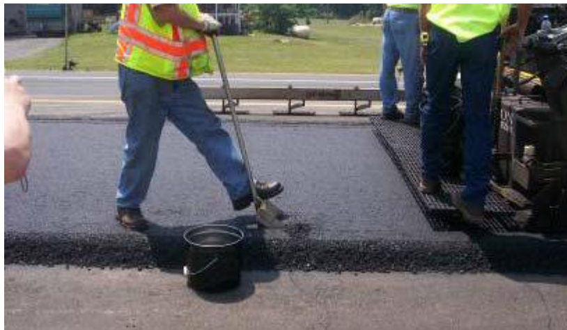
Figure 5-115 Shoveling material from above plates
