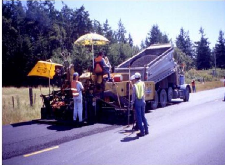
Figure 5-103: End dump of HMA into paver hopper (Mahoney, Pavement Interactive.com)
