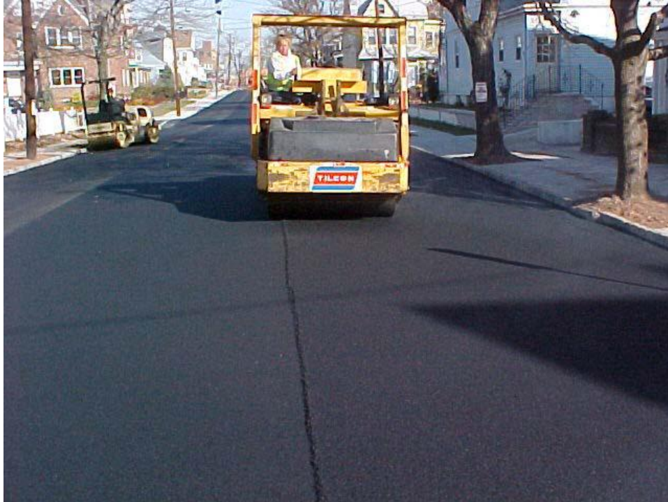
Figure 5-109: Rolling of hot mat for joint compaction (Benson and Scherocman 2006)
