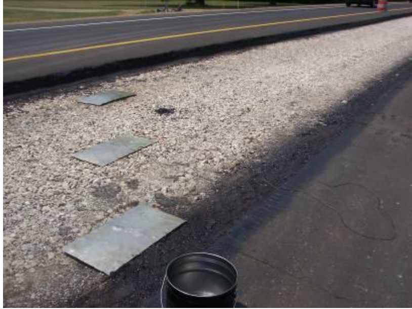
Figure 5-114 Plates randomly placed under HMA mat
