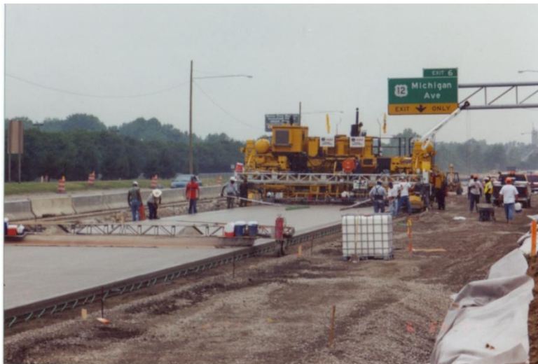
Figure 5-99: Quality construction is critical and contractor pay incentives are very helpful
