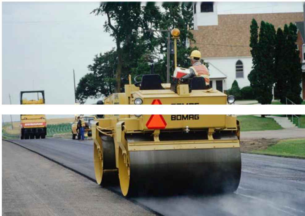
Figure 5-107: Proper rolling of free edge (Benson and Scherocman 2006)
