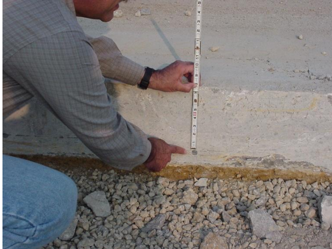
Figure 5-98: Tie bar placement is important and should be measured every day
