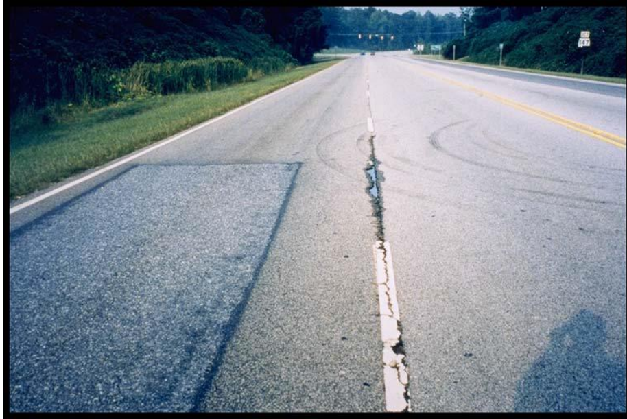
Figure 5-106: Raveled longitudinal joint (Brown, 2006)
