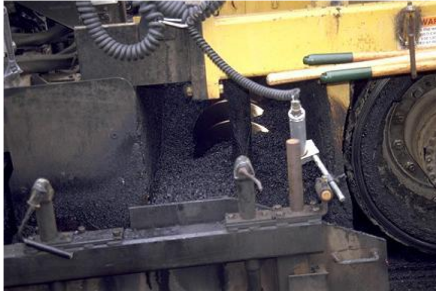
Figure 5-104: HMA head in auger (Mahoney, Pavement interactive.com)
