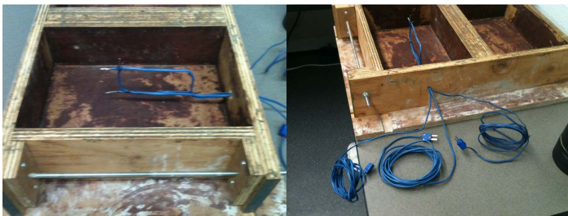
Figure 2. Thermocouples prior to concrete placement
