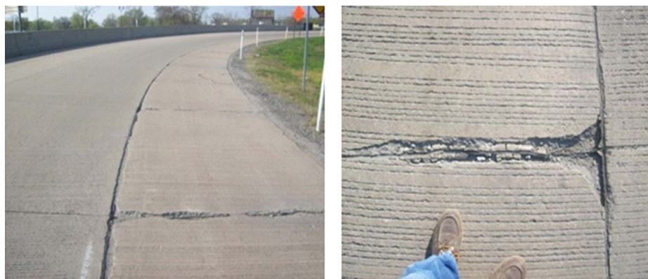
Fig. 1. Field observation showing damage in pavement joints
