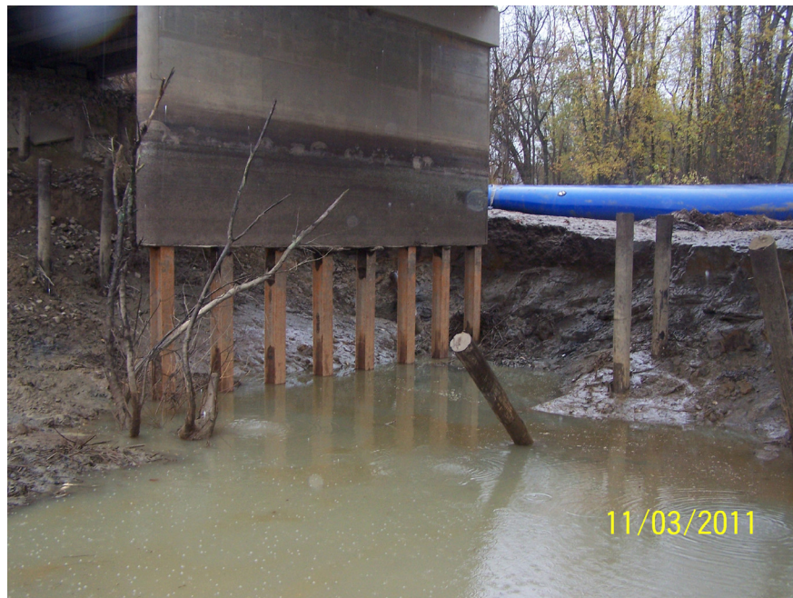
Figure 31. Photograph of bridge pier in Figure 30 taken after dewatering.
