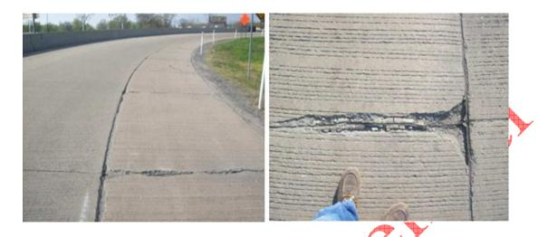
657 Fig. 1 Photograph of field observation showing damage in pavement joints
