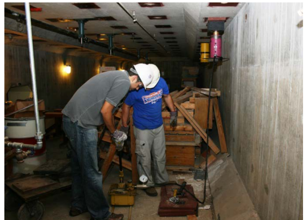
Fig. 4 Post-tensioning the column for the second 9-ft. test set-up
