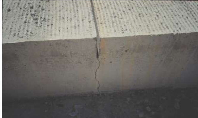
Figure 2.5 Aggregate interlocks [41]
