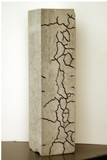
Figure 1. Example of freeze–thaw damage.
