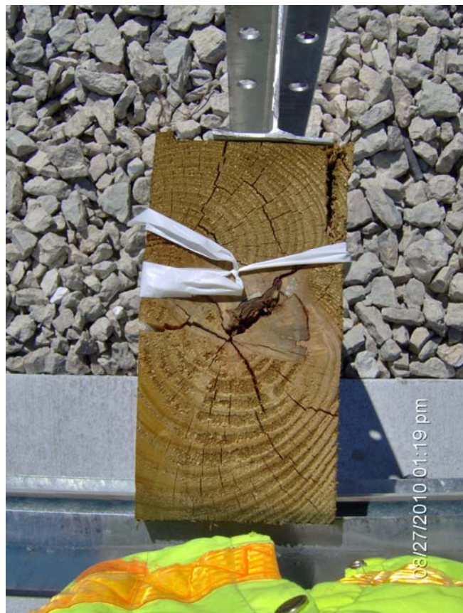
Figure 3. Wood Blockout Splitting
