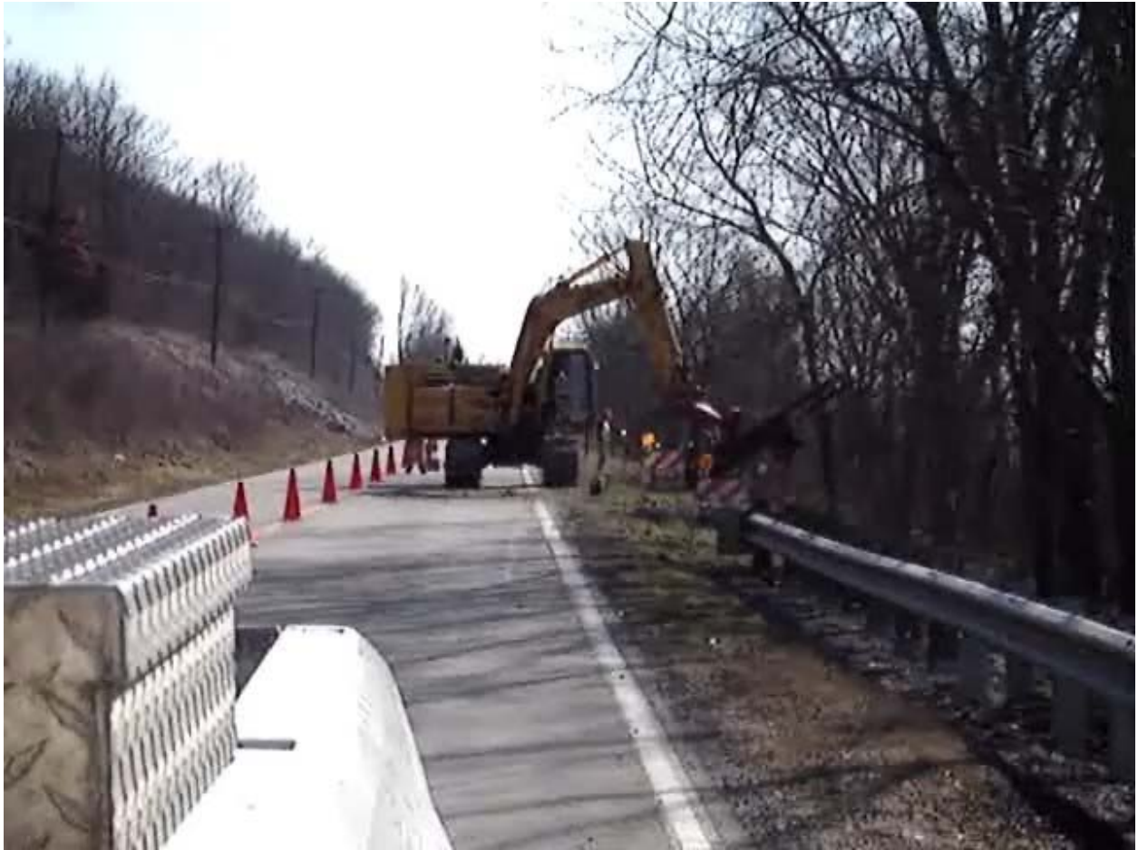
Figure 4. Guardrail Placement in an Cut Area
