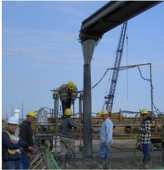
Fig. 5.14 – Typical conveyor drop for LC-HPC-11
