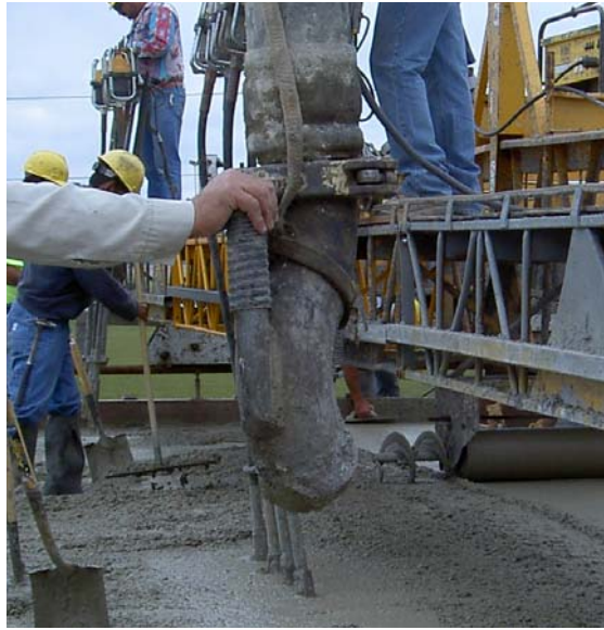
Fig. 5.12 – Elbow fitted to the end of the pump hose to limit air lose through the pump.
