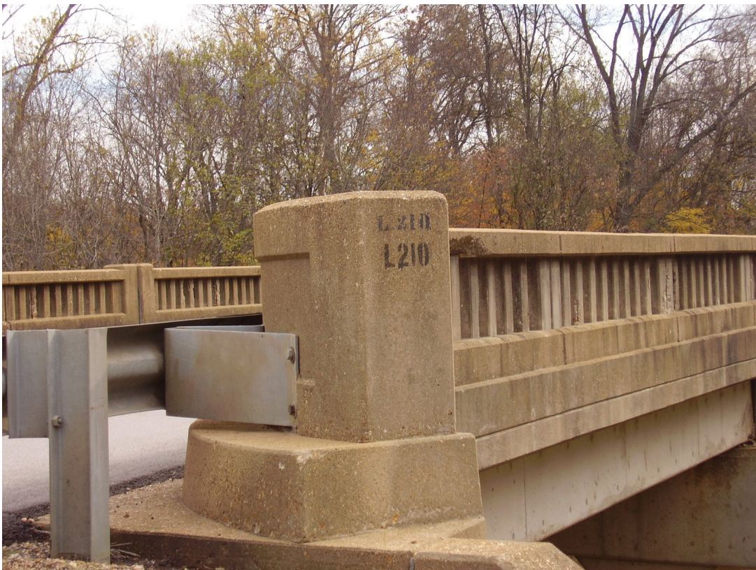
Figure 1. Curved Rail W-beam Transition
