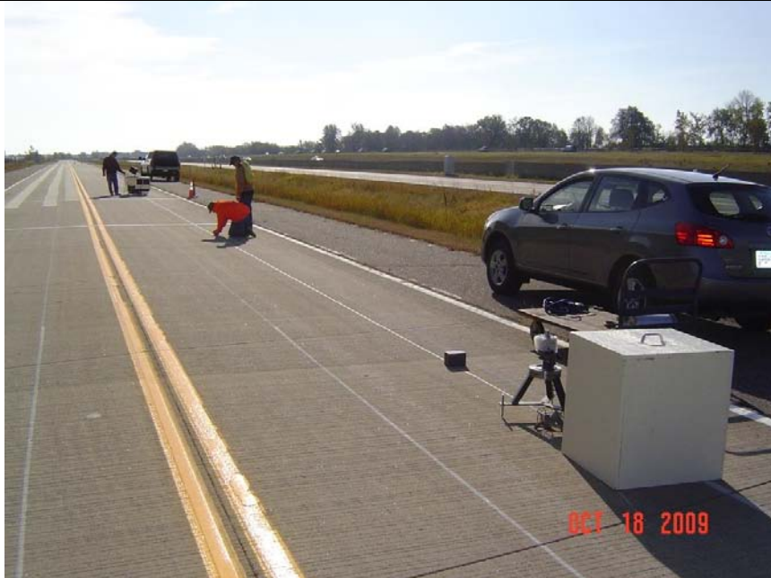
Benchmark Cart System Following Steel Tape
