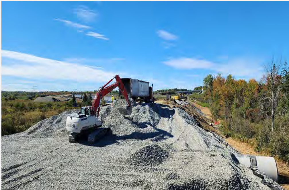
Delivery, Placement and Compaction of ULFGA
