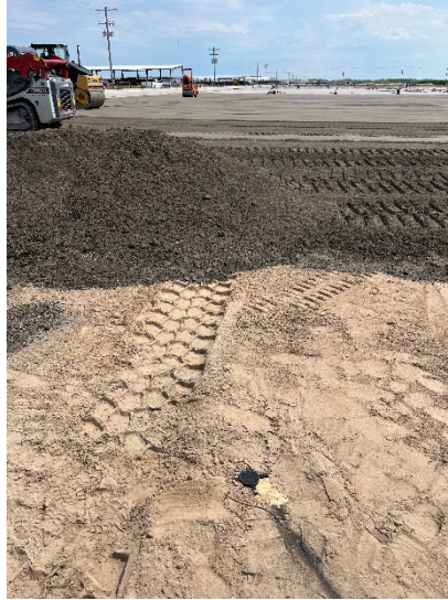
Figure 13. REBEL sensor in the roller-compacting concrete
