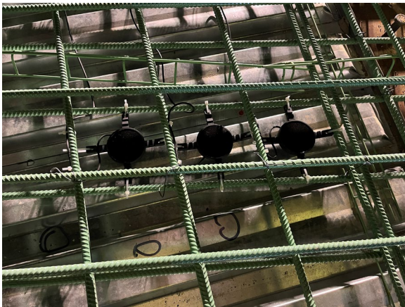
(a) Sensors were installed in the deck.
